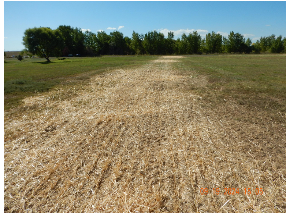
Photo 2. Photo taken from the well location, facing West. Photo illustrates final reclamation along the flowline path where the flowline has been removed.
