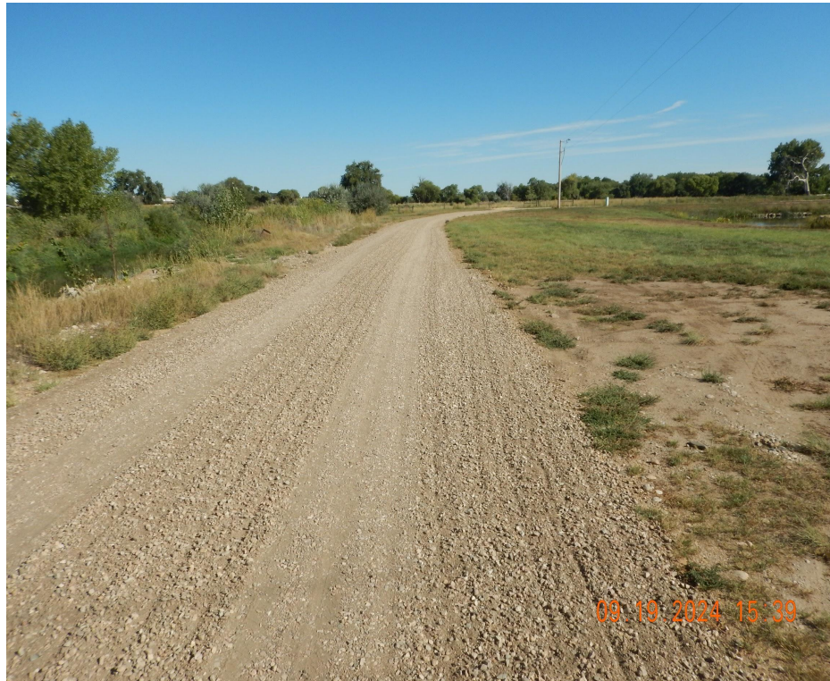
Photo 1. Photo taken from a southern portion of the access road, facing Southeast. Photo illustrates Operator has completed repair road damages by importing surface owner approved gravel.
