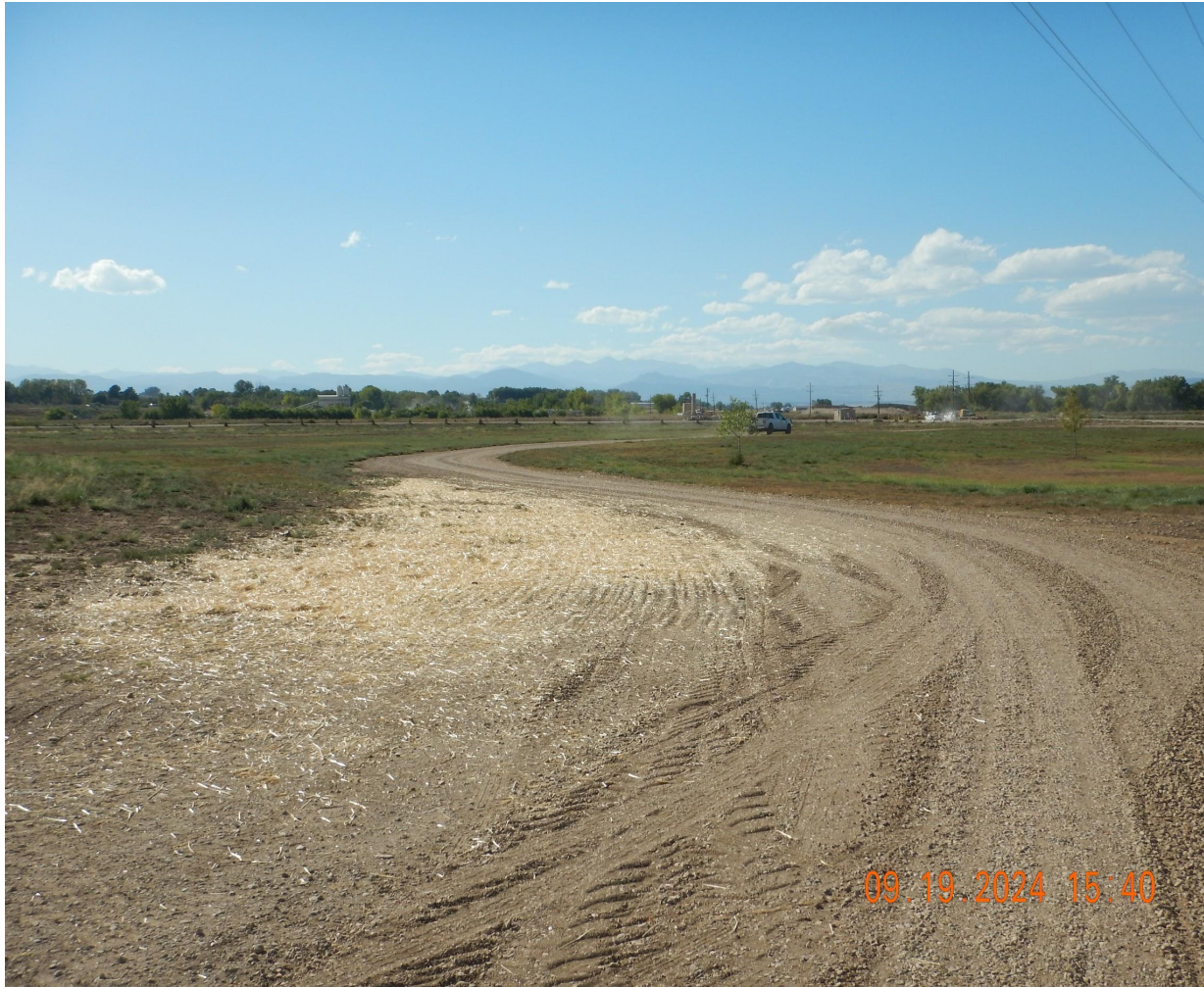
Photo 3. Photo taken from a central portion of the access road, facing Northwest. Photo illustrates Operator has completed repair road damages by importing surface owner approved gravel and seeded/straw crimped mulch to reduce road surface disturbances.
