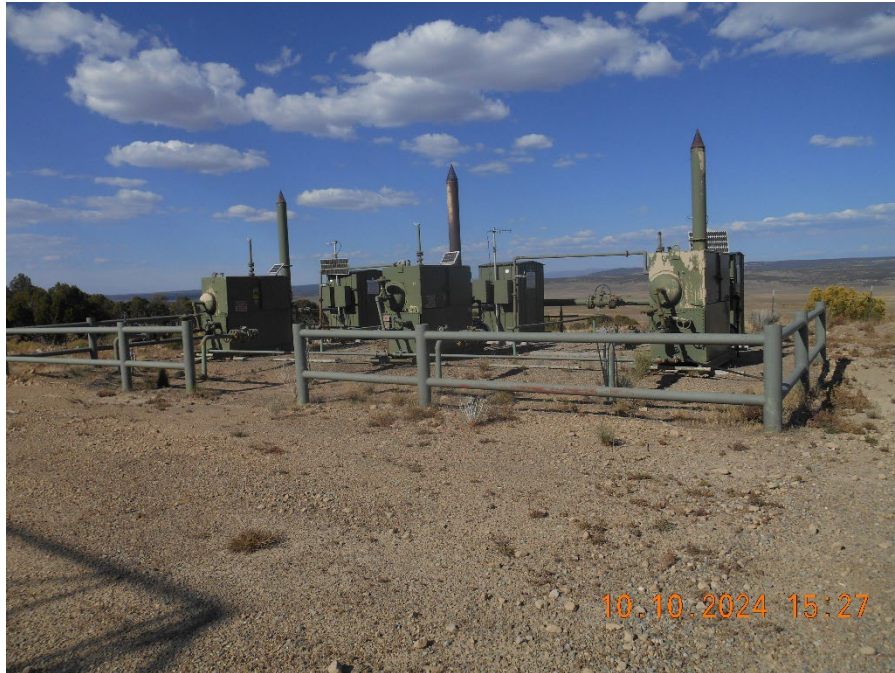
Separators and Meter housings
