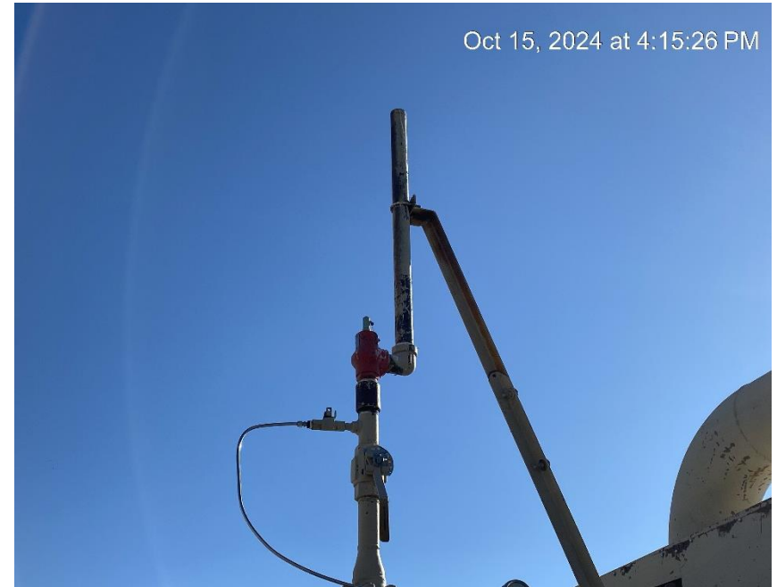
Relief vent riser missing cap
