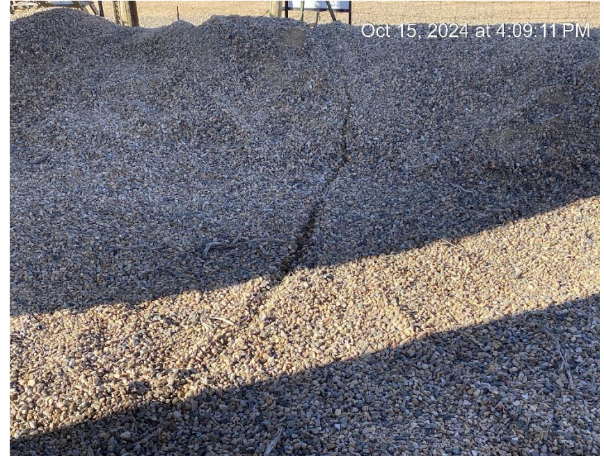
Staining from hose dragging
