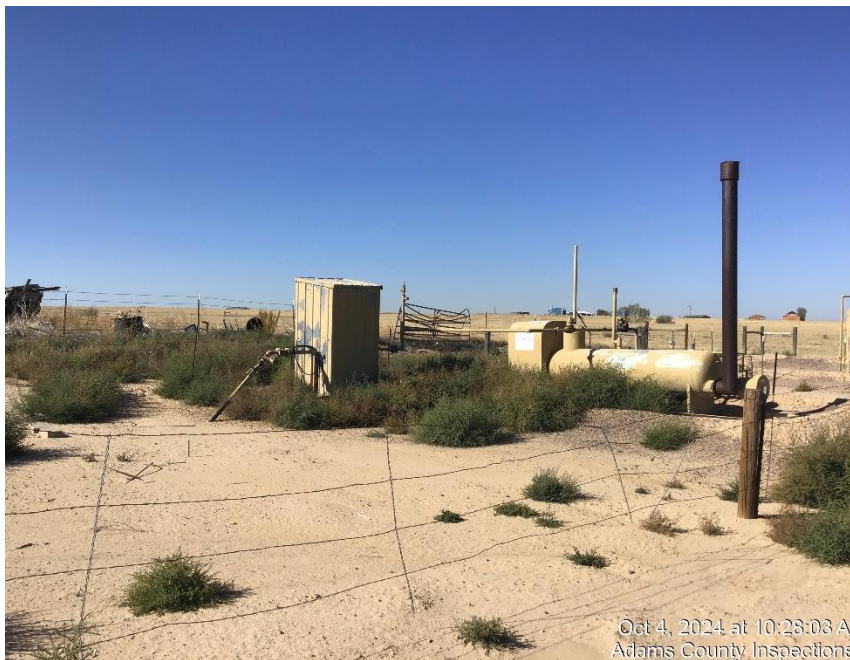
Photo #5 Meter run and Separator (weeds throughout location)
