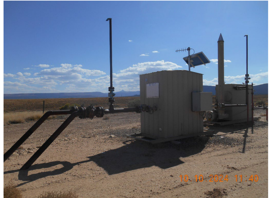
Separator and Meter housing
