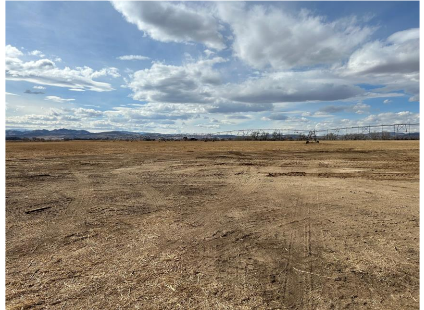
Well 20-3 Well pad after backfilling prior to seeding.
