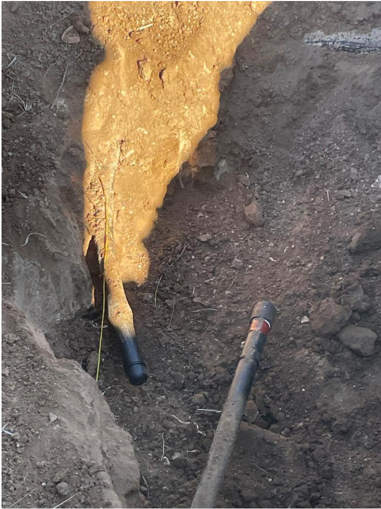
Well 20-3 Flowline separation and capping at trunk line.
