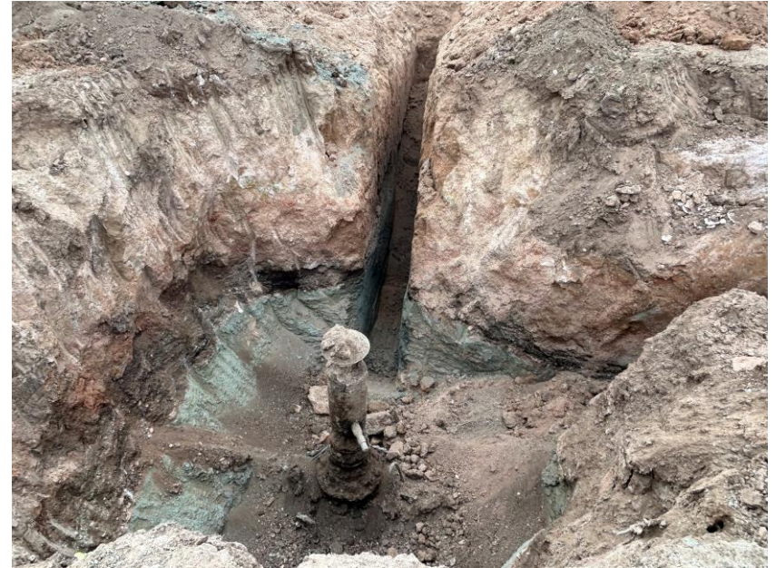
Well 20-3 Wellhead excavation looking west.
