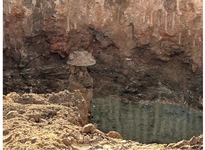
Well 20-3 Wellhead excavation looking south at petroleum contamination, (dark layer on top of weathered shale).
