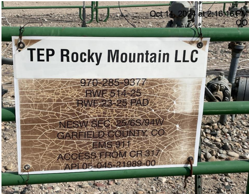
Photo # 5336 Wellhead sign weathered & cracking
