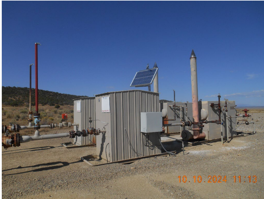
Separators and Meter housings
