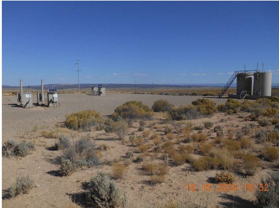
Location overview looking N
