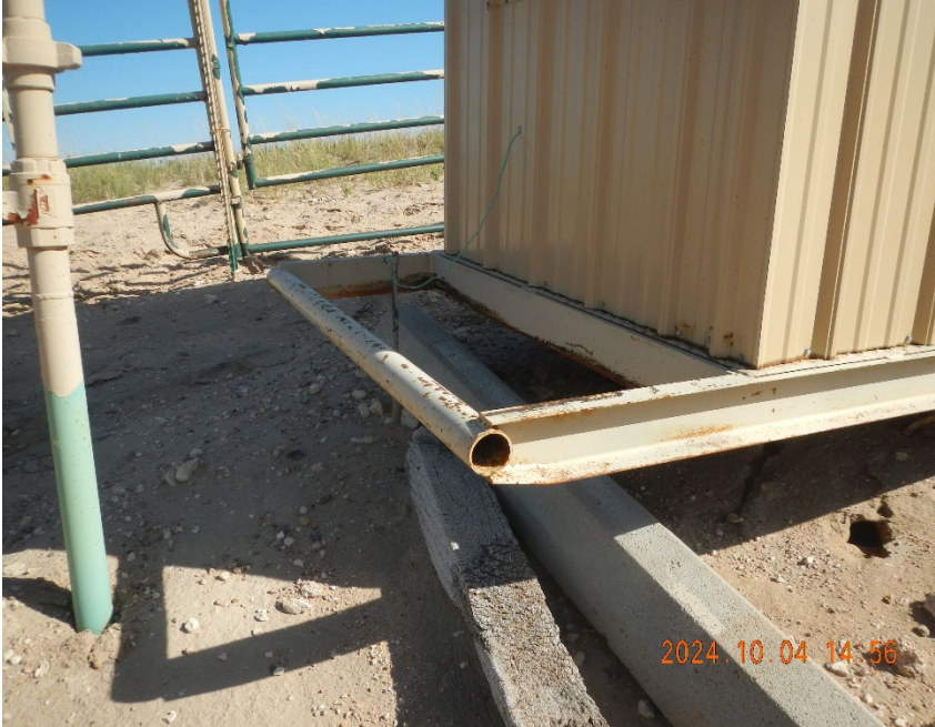
5. View of meter shed off footer and cribbing.
