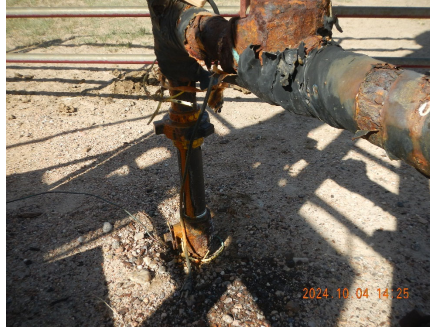
4. View of water leg hammer union
