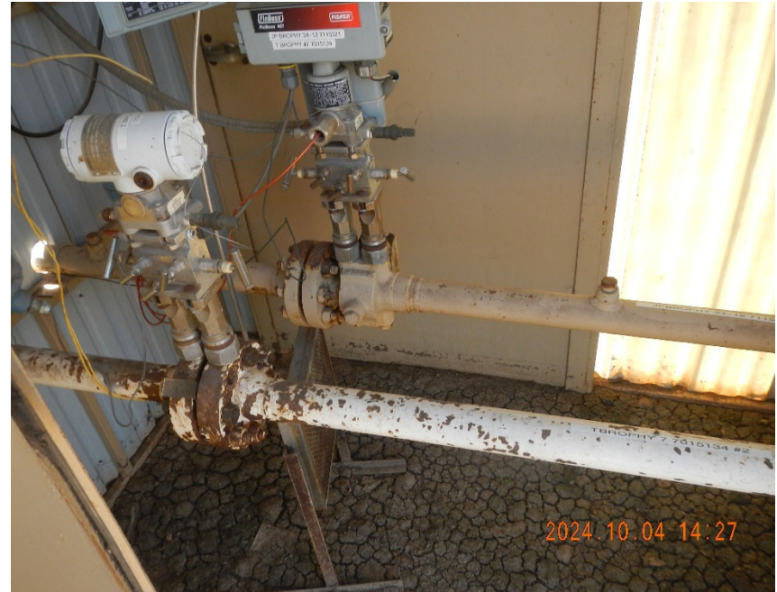
6. Gas meter inside shared meter shed.
