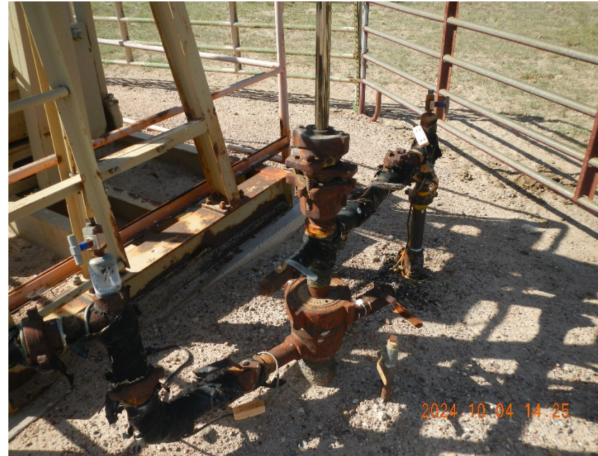
2. View of wellhead. Active release at water lag hammer union.
