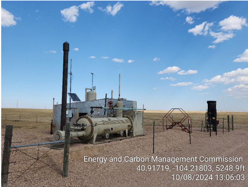
Photo 3 – Separator and ECD
