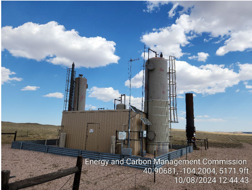
Photo 3 – Heater Treaters and ECD
