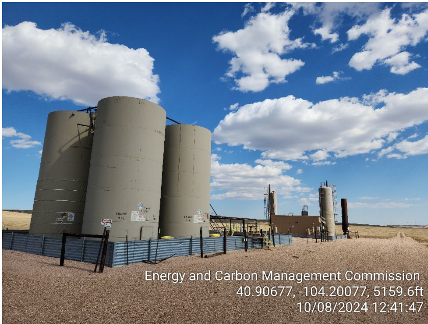
Photo 1 – Tank Battery
