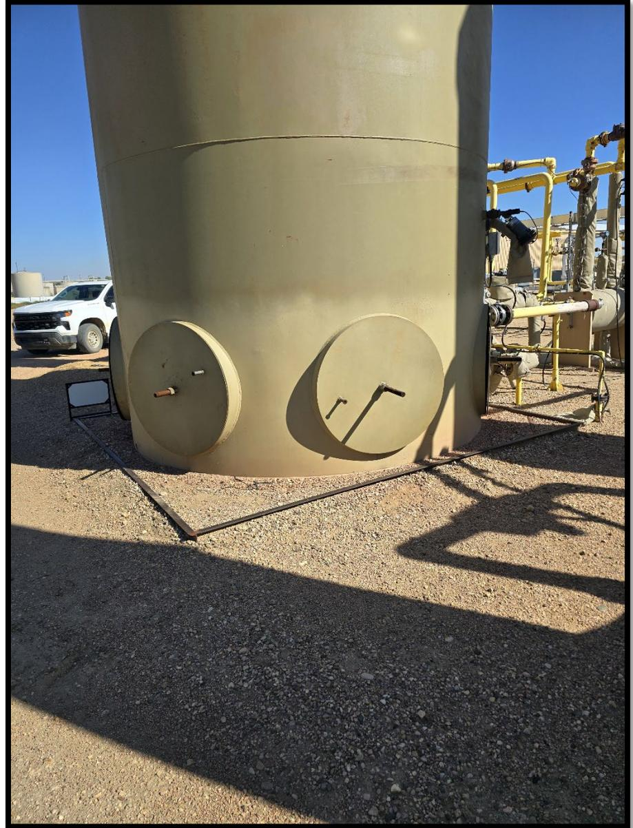
**CA:** Install wildlife screens on separator #10, see attached photo. Install wildlife screen per Rule 608.b.(7).
