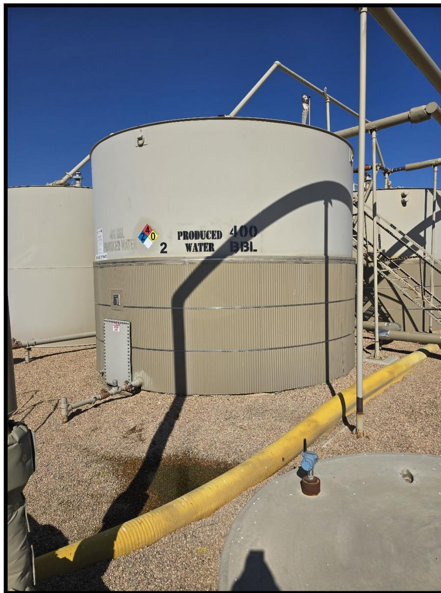
**CA:** North row of 400 bbl crude oil tanks and both 400 bbl produced water tanks contents and capacity placards have faded and are illegible, see attached photos. Install sign to comply with Rule 605.h.
