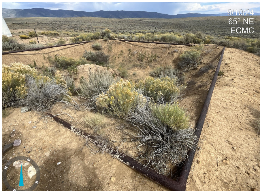
Photo 5. Photo taken from the southeastern pad surface, facing northeast. Photo illustrates insufficient or missing BMPs on pit. Operator shall install/maintain stormwater BMPs per Rule 1002.f.(2)
