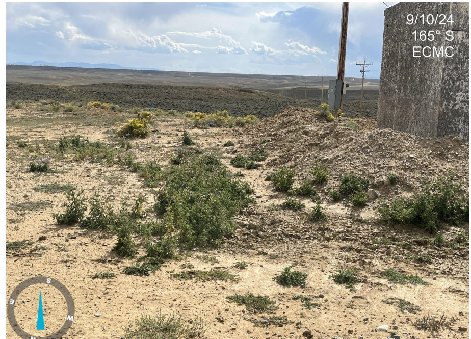
Photo 2. Photo taken the entrance of the Location, facing south. Weeds observed growing along the perimeter. Photo illustrates failure of stormwater BMPs. Operator shall repair stormwater BMPs per Rule 1002 and control weeds per Rule 606.
