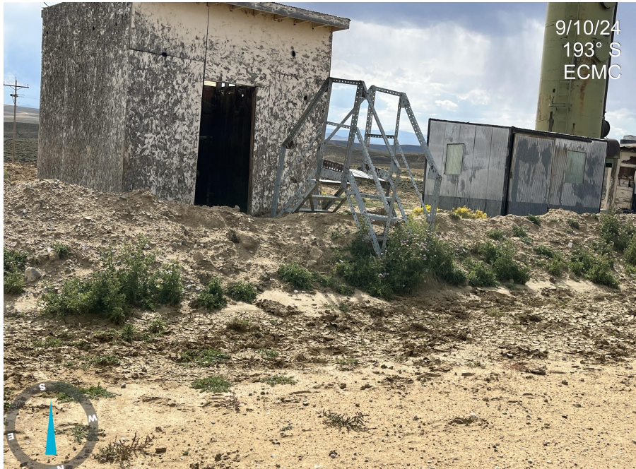
Photo 3. Photo taken from the pad center, facing south. Photo illustrates weeds growing in secondary containment berms. Secondary containment does not appear to be adequate. Comply with Rule 1002.f.(2). and 606.c.
