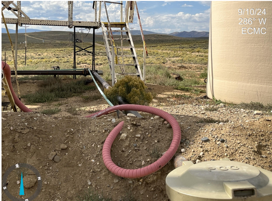
Photo 8. Photo taken from the western pad surface, facing west. Photo illustrates a hose which could contribute to a potential spill if not connected, capped, and stored in secondary containment.
