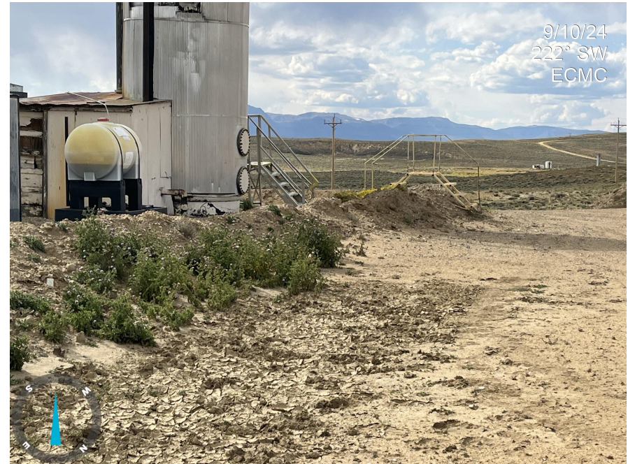
Photo 4. Photo taken from the pad center, facing southwest. Photo illustrates failing BMPs and weeds. Comply with Rule 1002.f.(2). and 606.c.
