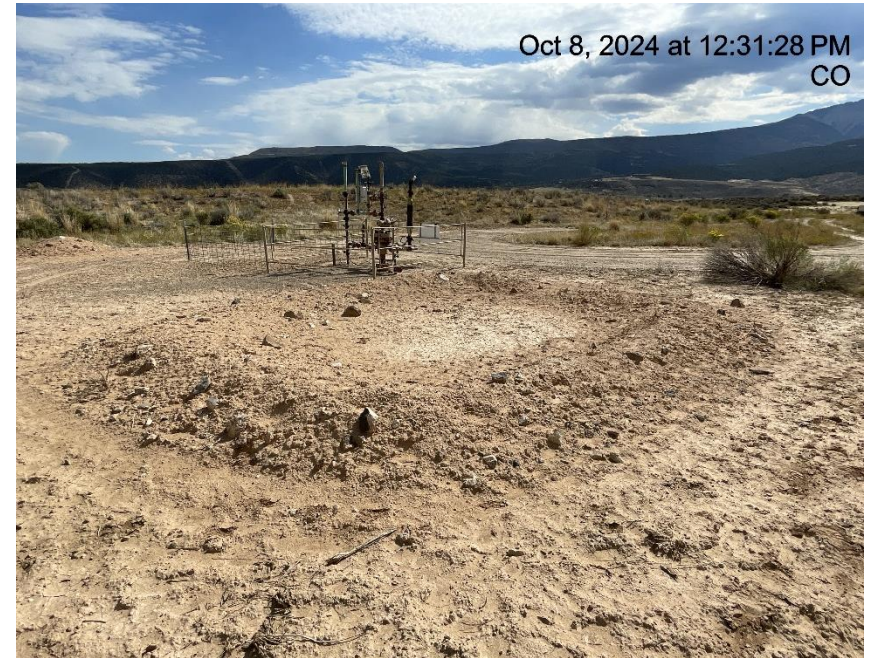
Photo # 4030 Unused dirt berm containment
