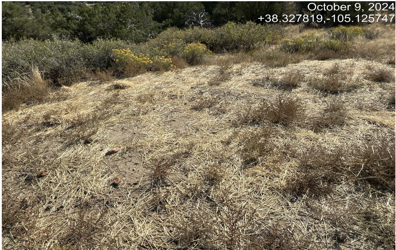
Photo 2. The straw mulch was not crimped and soils may not be still seem compacted. This would impact revegetation.
