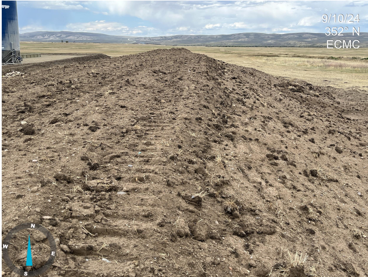
Photo 15. Photo taken on top of topsoil stockpile. It was observed that temporary stabilization/roughening was implemented.
