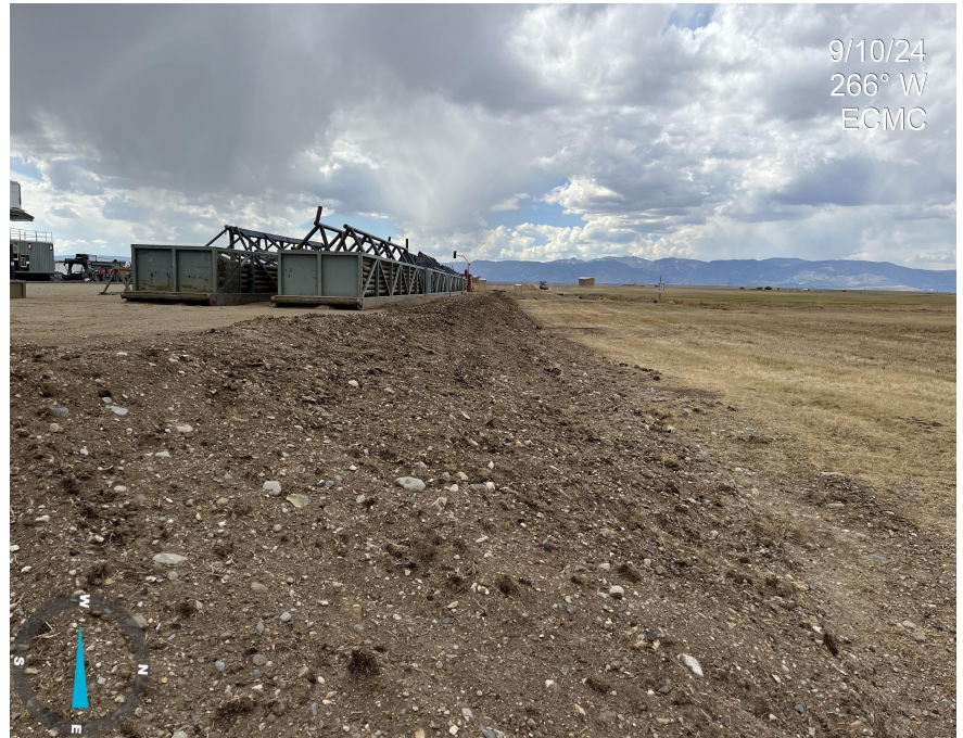
Photo 8. Photo taken from the northeastern edge of Location, facing west. Photo illustrates perimeter stormwater BMP.
