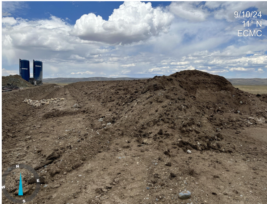
Photo 13. Photo taken on eastern edge of Location. Photo illustrates topsoil stockpile. It was observed that the topsoil was temporarily tracked. No other BMPs have been implement in conjunction with tracking to minimize erosion, degradation and sediment transport per good engineering practices.
