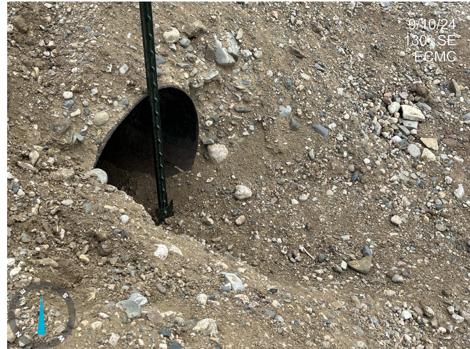
Photo 10. Photo taken from entrance of Location, facing SE (i.e., other side of road). Photo illustrates culvert with no inlet/outlet protection.
