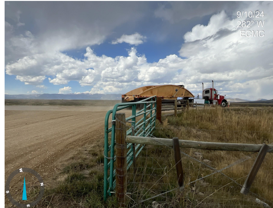
Photo 4. Photo taken from the entrance of access road Location facing Highway 14. Tracking pad not installed to prevent track of material off site. Discussion with Operator that street sweeper was employed to clean sediment tracked off-site.
