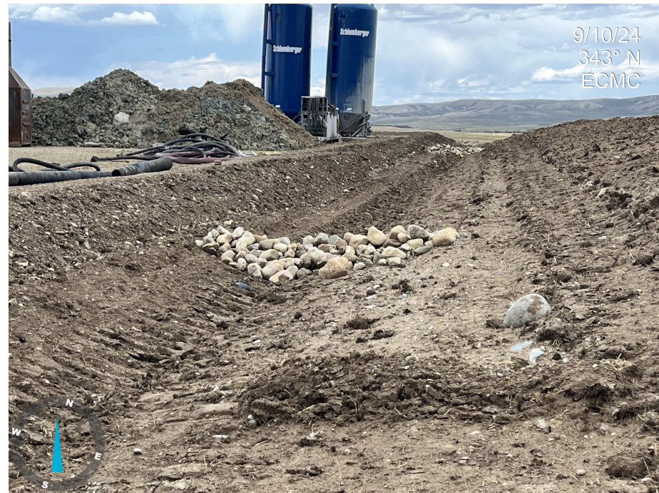
Photo 12. Photo taken from the eastern edge of Location. Photo illustrates check dams in perimeter ditch.
