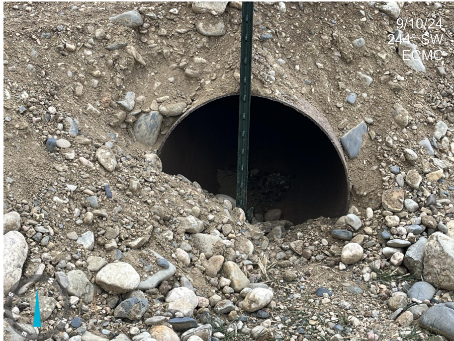
Photo 9. Photo taken from entrance of Location, facing SW. Photo illustrates culvert with no inlet/outlet protection.
