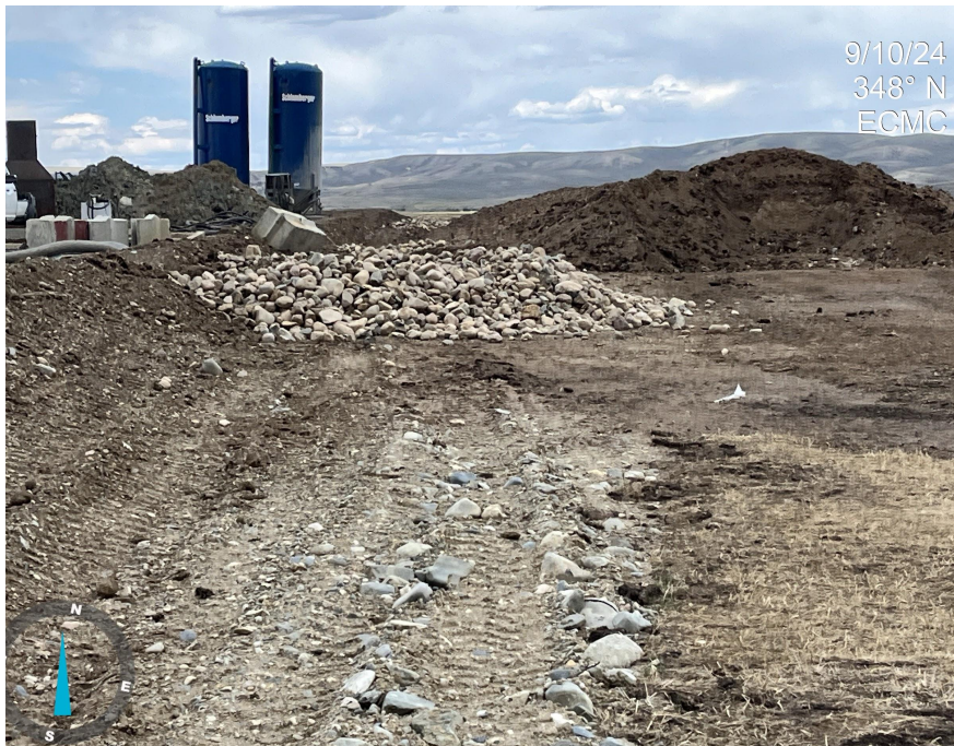
Photo 7. Photo taken from the southeastern edge of Location, facing north. Photo illustrates perimeter stormwater BMP, stormwater outlet, and topsoil stockpile.
