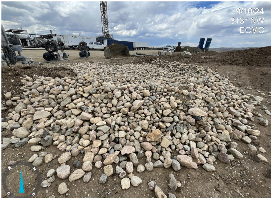
Photo 11. Photo taken from the eastern edge of Location.. Photo illustrates stormwater outlet. It was observed that round river rock was implemented not per good engineering practices.
