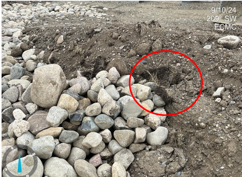
Photo 16. Photo taken on eastern edge of Location. Photo illustrates topsoil was used in sediment trap. Utilization of topsoil material as part of stormwater controls does not comport with Rule 1002.c, as this places the topsoil resource at risk to degradation, contamination (commingling with sediment), and loss of the resource.
