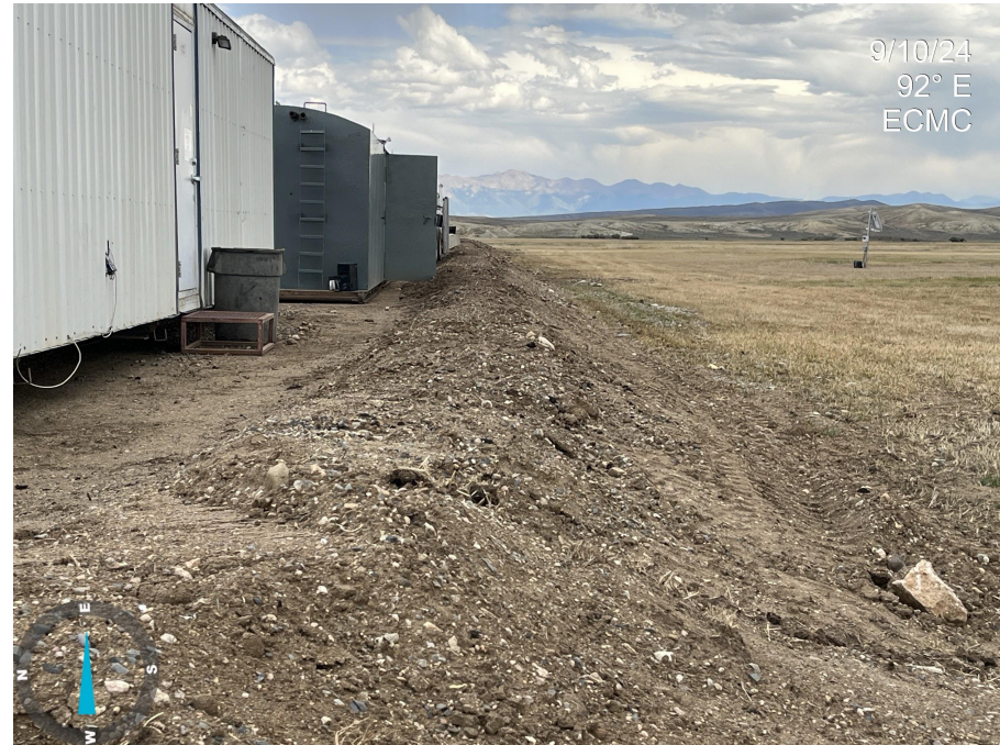
Photo 6. Photo taken from the southwestern edge of Location, facing east. Photo illustrates perimeter stormwater BMPs.
