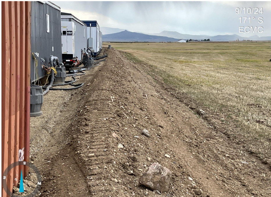
Photo 5. Photo taken from the northwestern edge of Location, facing south. Photo illustrates perimeter stormwater BMPs.
