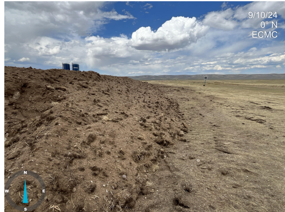
Photo 14. Photo taken on eastern edge of Location. Photo illustrates topsoil stockpile with no perimeter stormwater BMPs. Operator shall implement topsoil stormwater BMPs per Rule 1002.f.(2).
