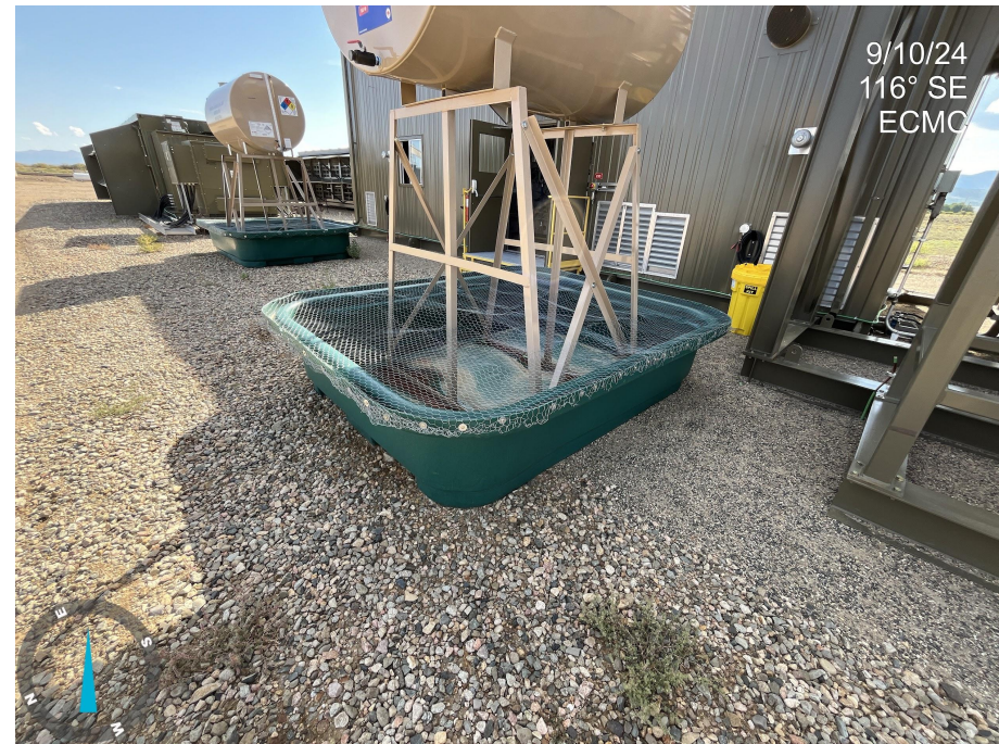
Photo 9. Photo taken from the southern working pad, facing SE. Photo illustrates that wildlife BMPs were implemented on secondary containment.
