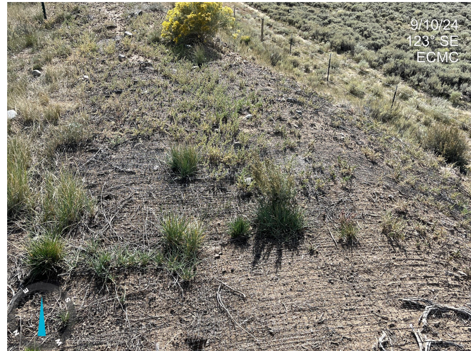
Photo 7. Photo taken from the eastern working pad, facing SE. Photo illustrates a portion of the topsoil stockpile with temporary BMPs (erosion control netting). Operator shall continue to monitor and manage until Location reaches 1002 standards.
