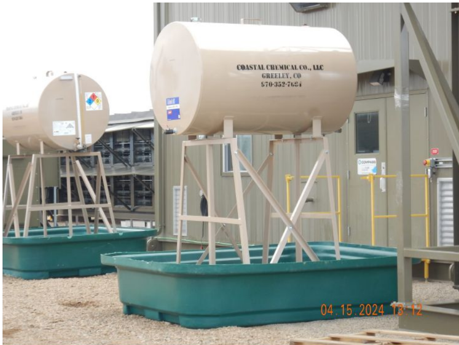
Photo 8. Photo taken 4/15/2024 from the southern working pad surface, facing Southeast. Photo illustrates the equipment and secondary containment lacks wildlife protection.
