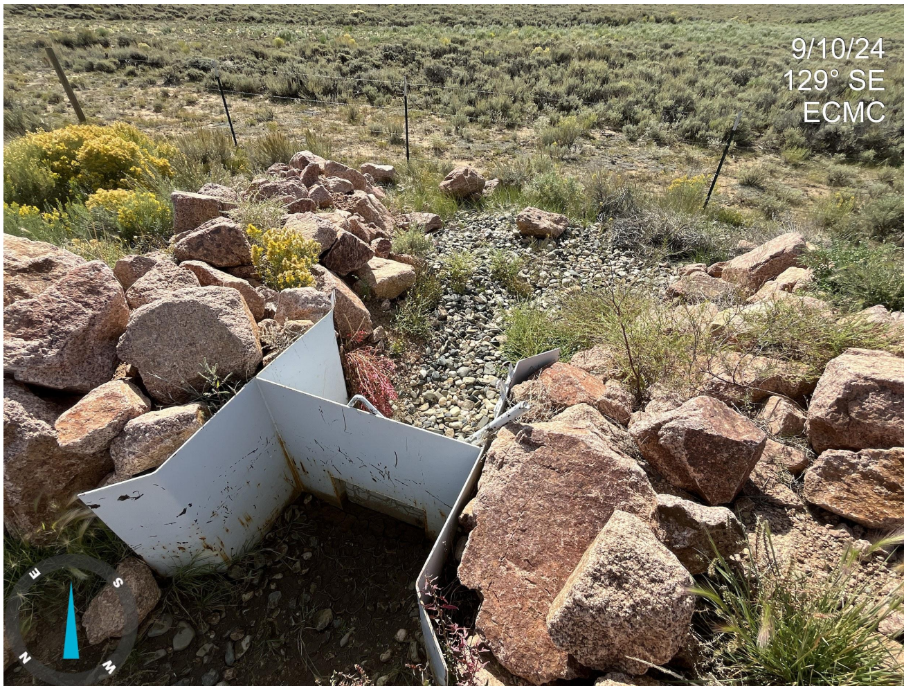
Photo 5. Photo taken from the southern working pad surface, facing SE. Photo illustrates the stabilized outlet. At the time of this inspection, there was no sediment discharge off of the Location.
