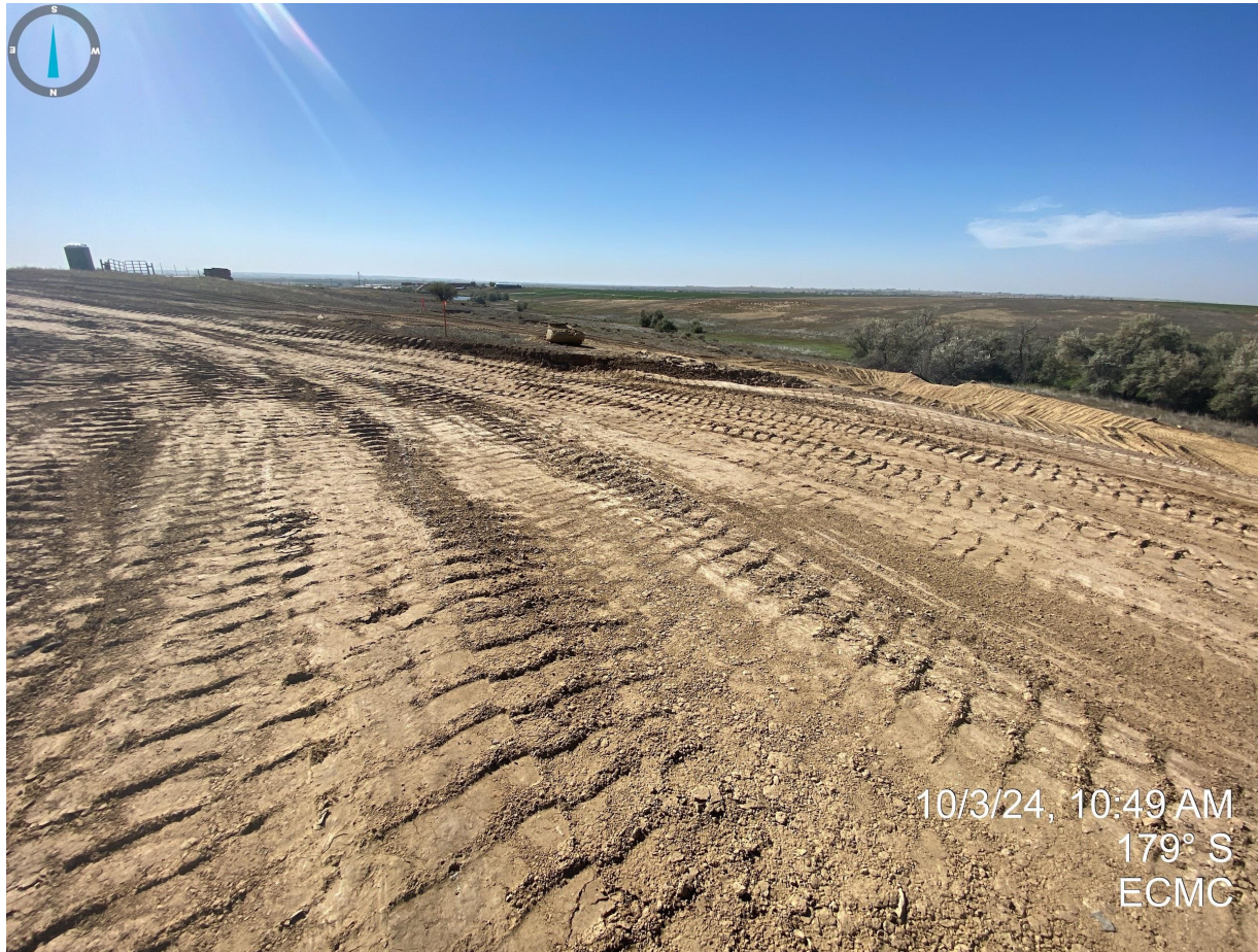
Photo 3. Facing south; see comments in Photo 1.
