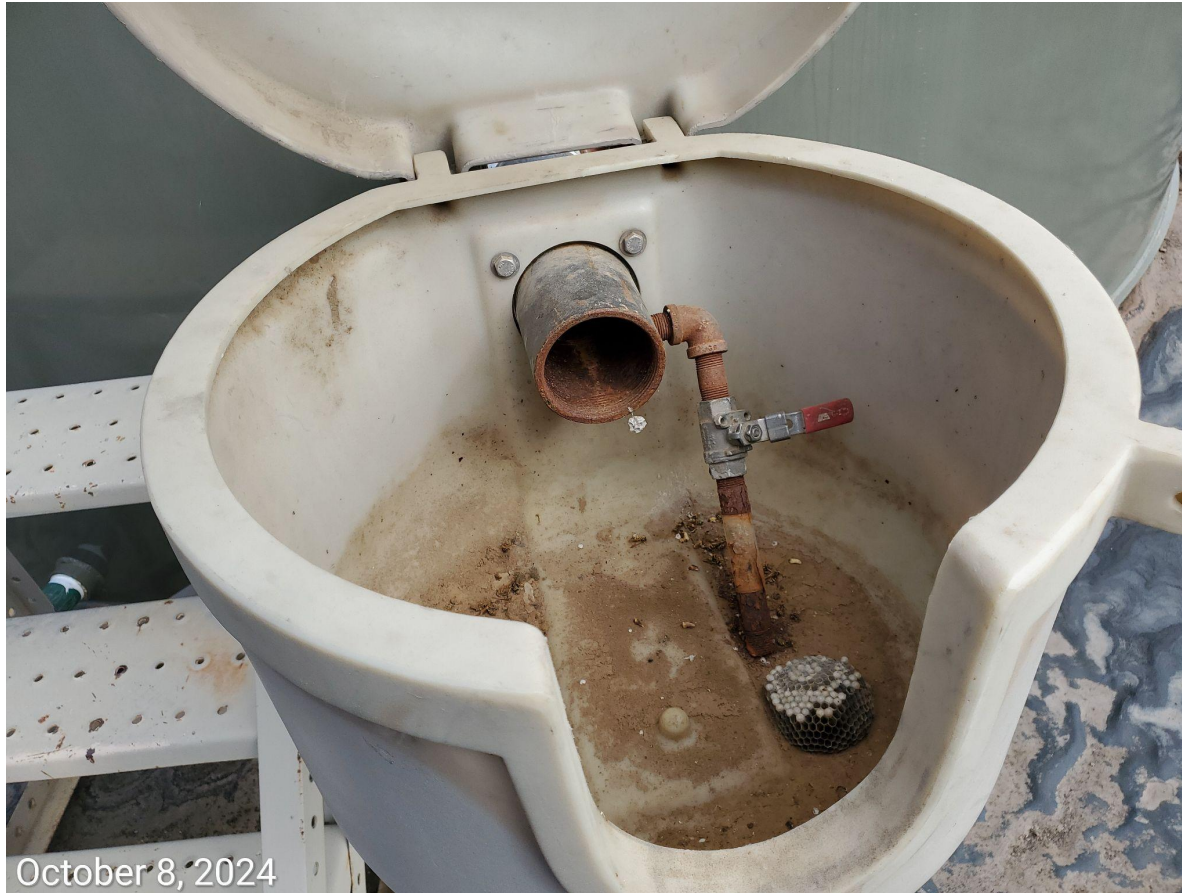
Photo 4: Line at tank missing cap/plug.
