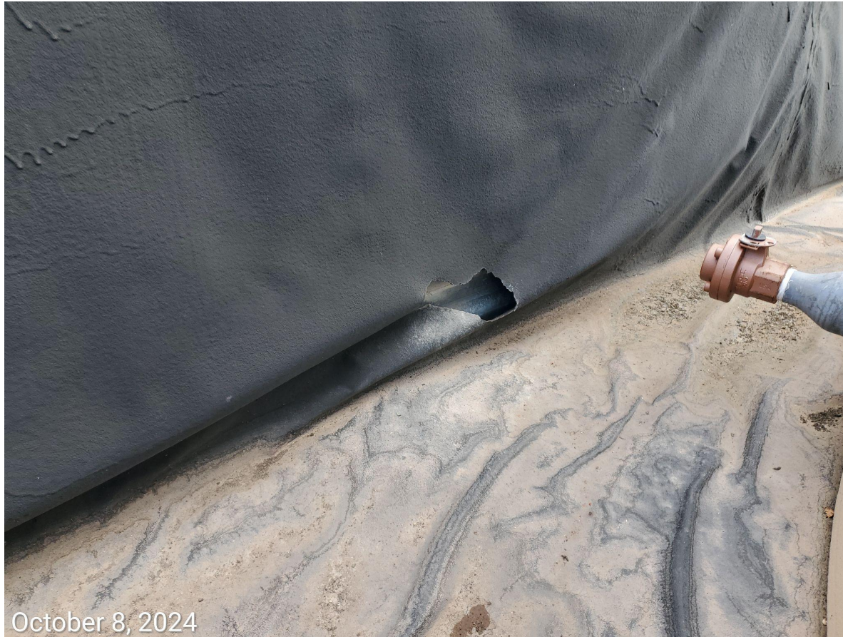
Photo 5: Photo taken from the tank battery facility's secondary containment BMP- BMP no longer sufficiently impervious to contain a spill or release.
