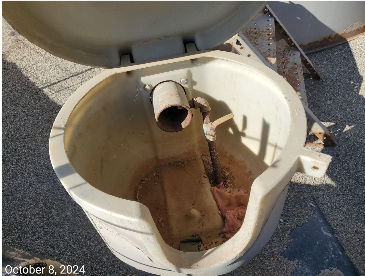
Photo 4: Line at tank missing cap/plug.
