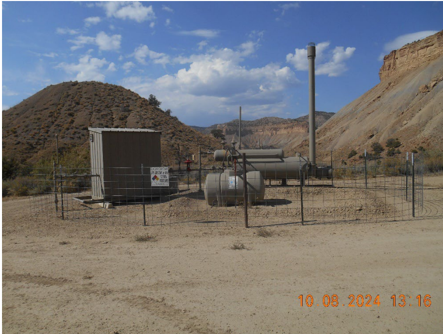
Separator and Meter housing
