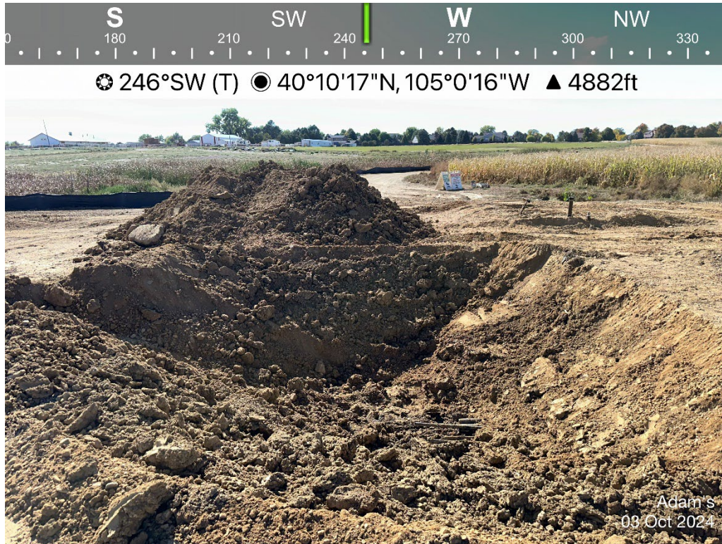
Tank Battery Excavation
