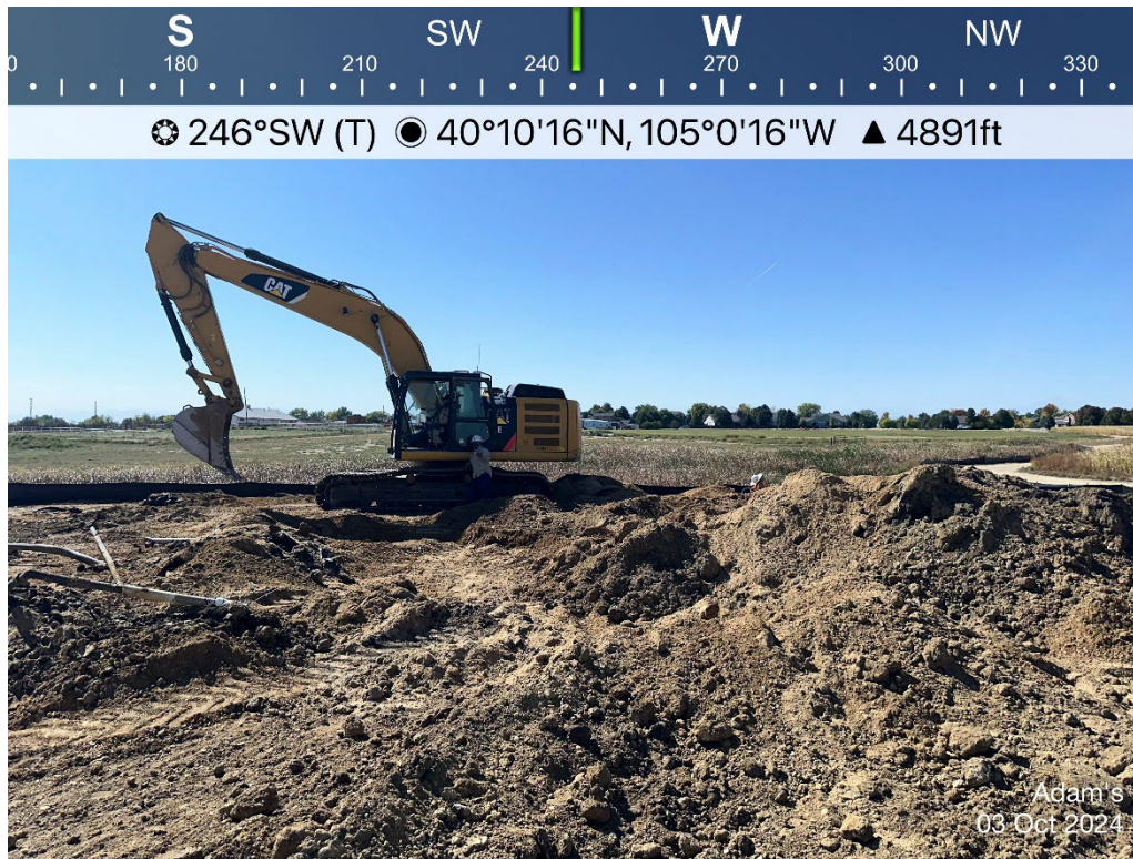
Tank Battery Excavation
