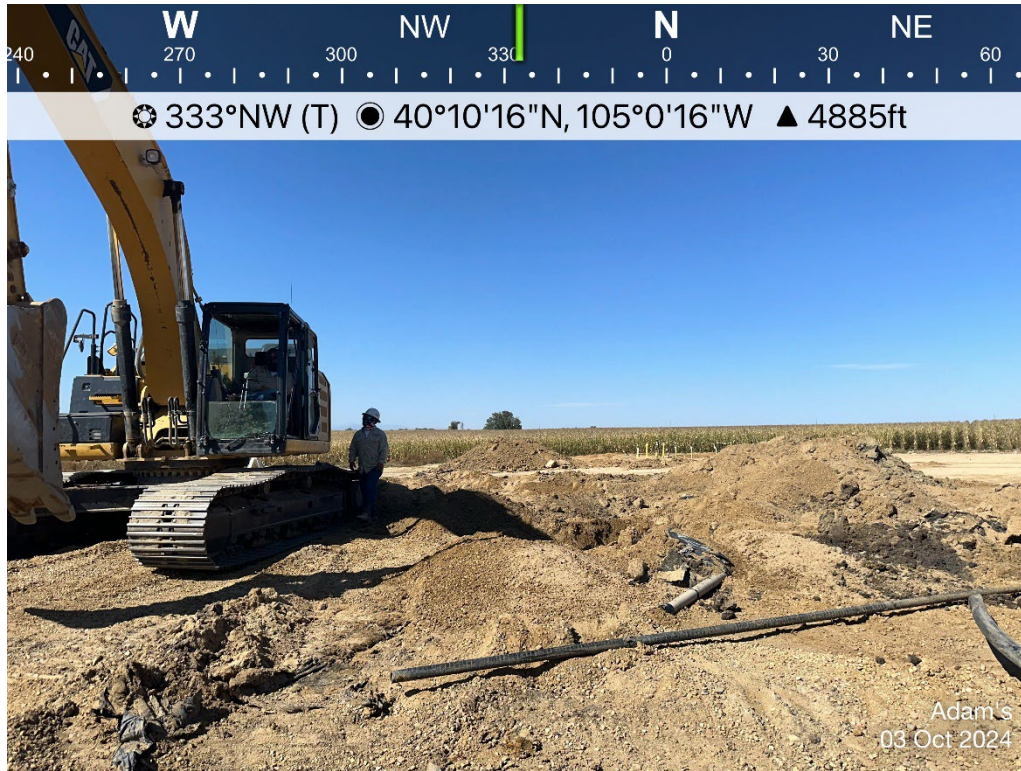
Tank Battery Excavation
