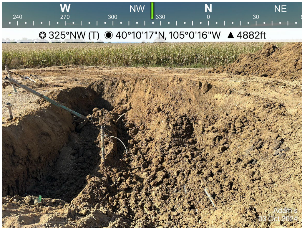
Tank Battery Excavation
