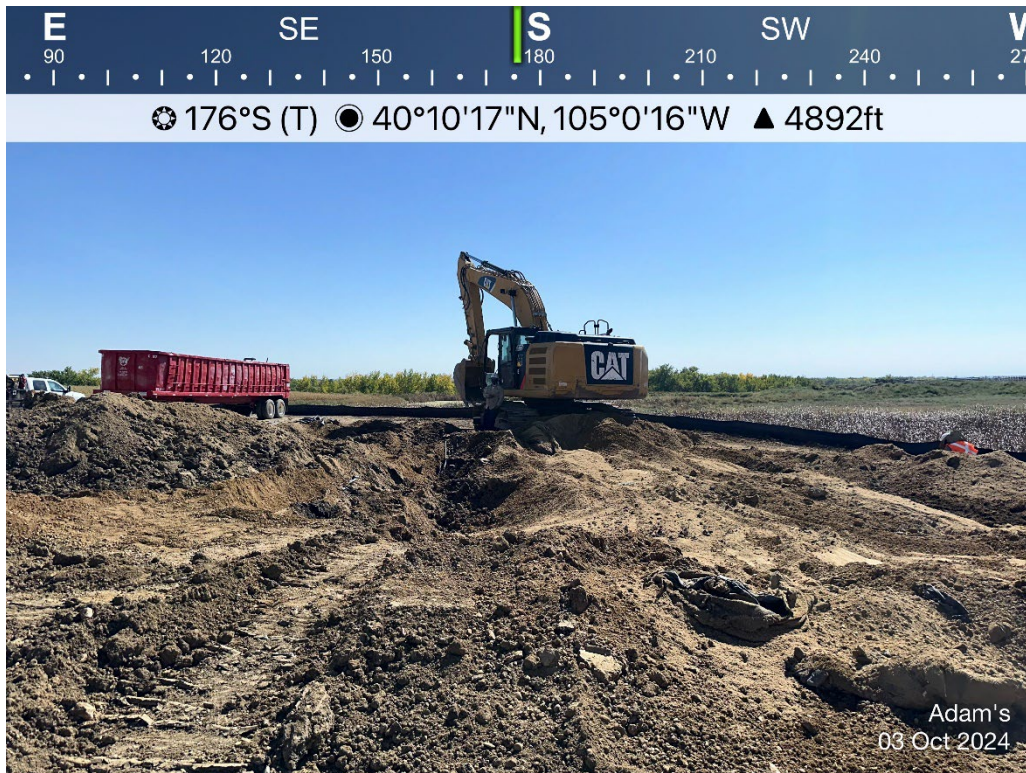
Tank Battery Excavation
