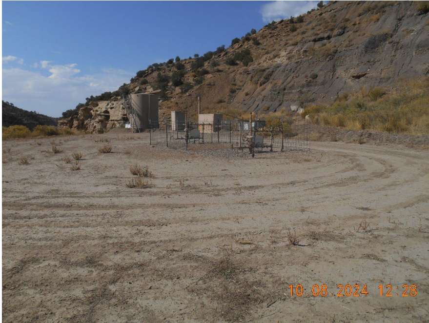
Location overview looking SW
