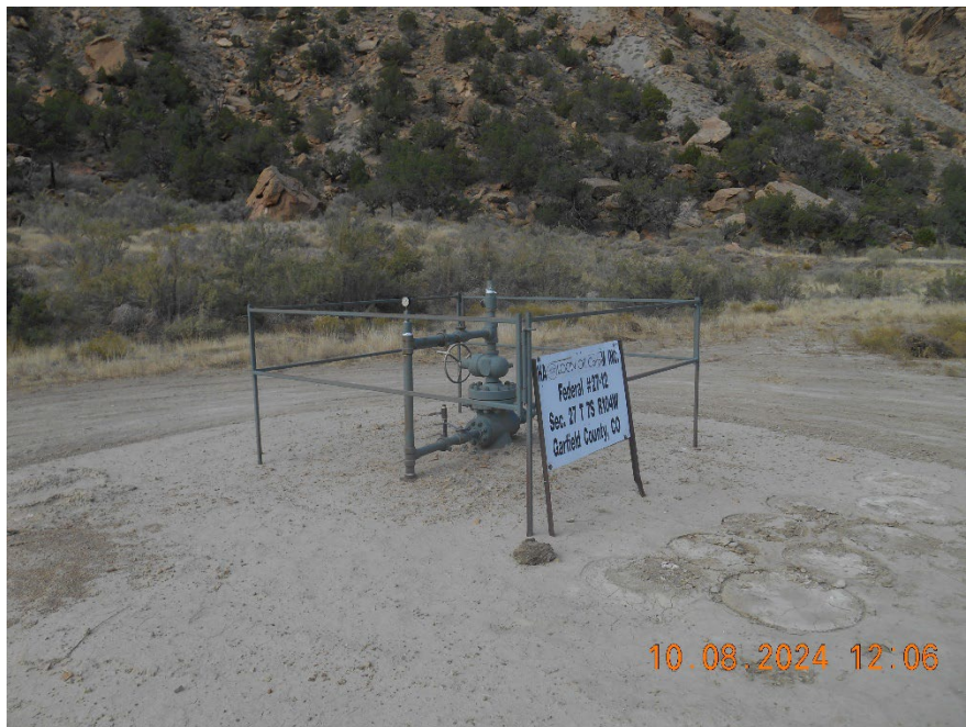
Wellhead with fence and sign
