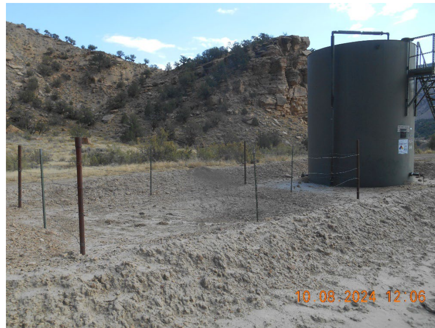
Tank battery. Blowdown tank removed.
