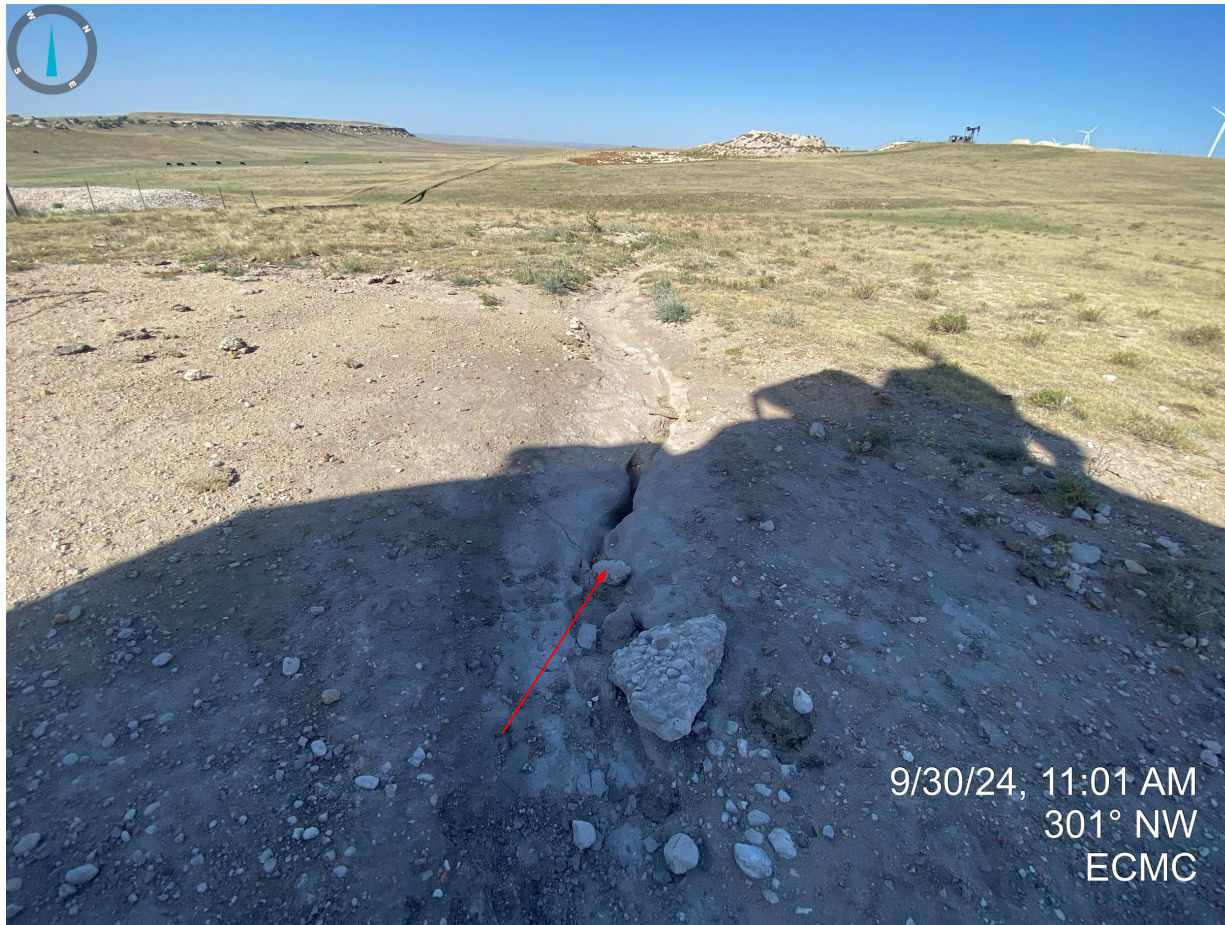
Photo 11. Erosion degradation observed on northside of meter shed.
