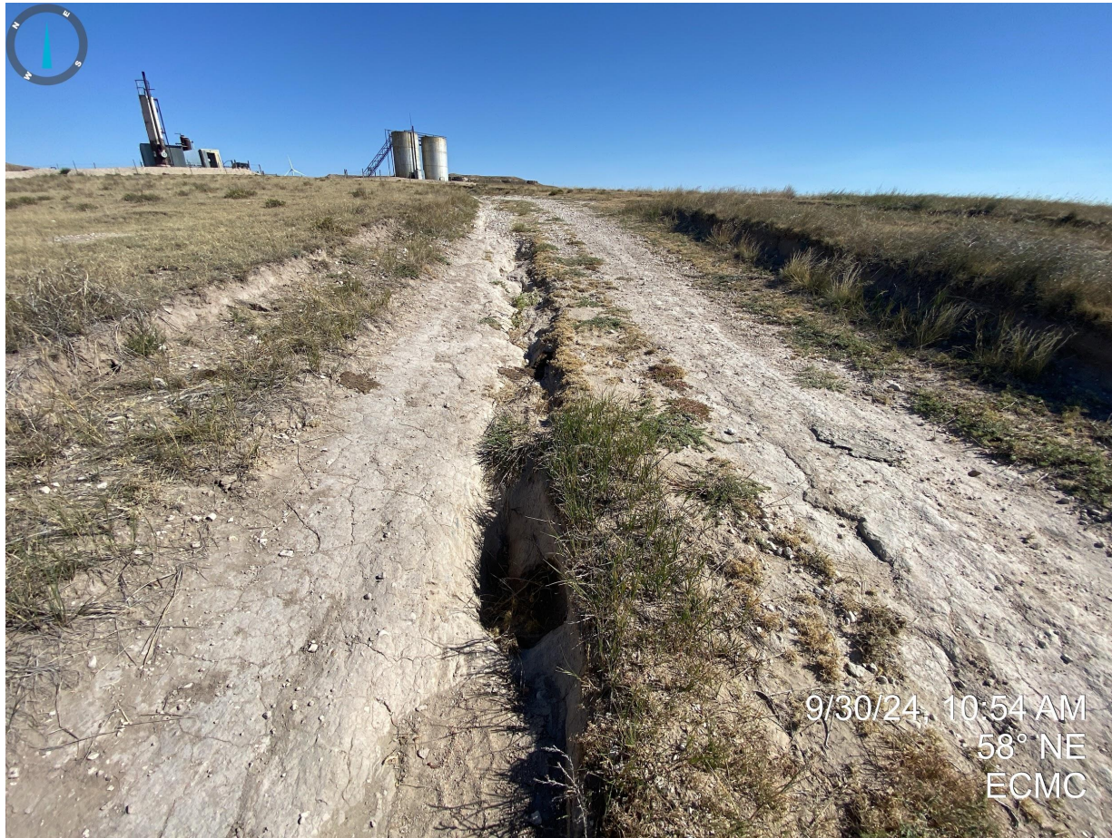
Photo 1. Erosion degradation south of the production facilities.
