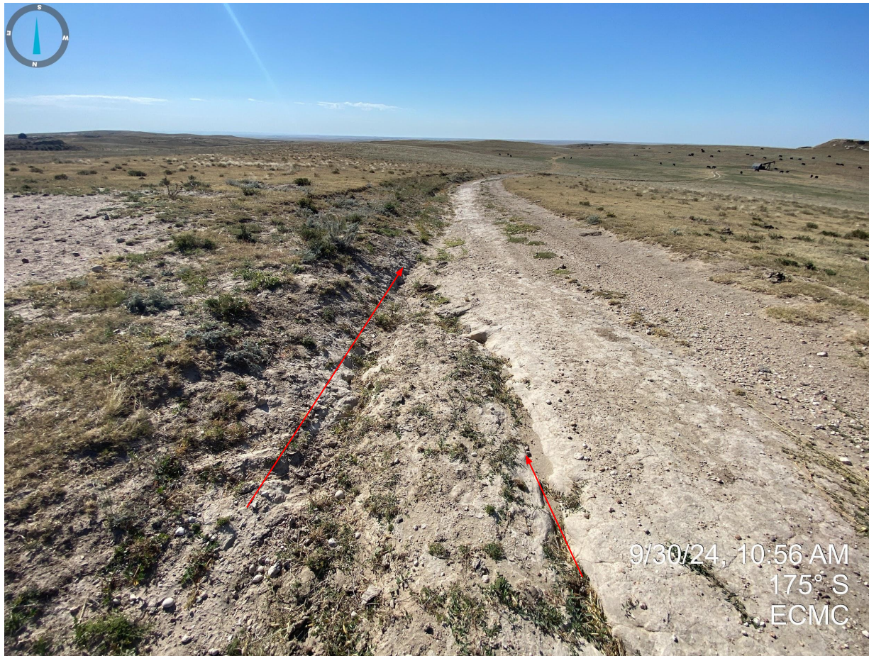
Photo 2. Erosion degradation south of the production facilities.
