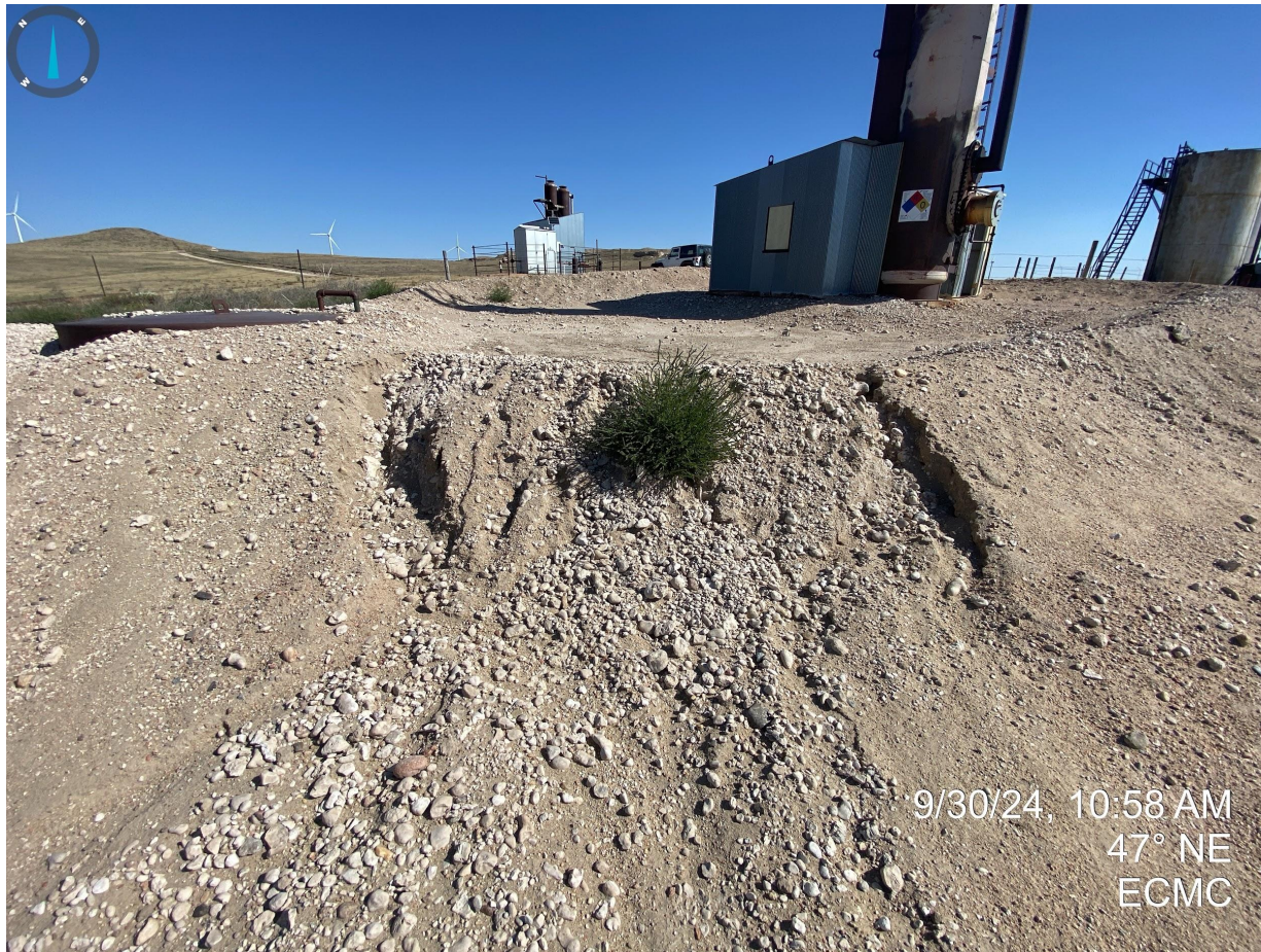
Photo 4. Undesirable vegetation and erosion degradation observed within the pit berm area.
