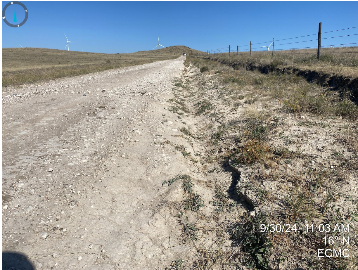
Photo 14. Erosion degradation observed along the access road, north of the production facilities.
