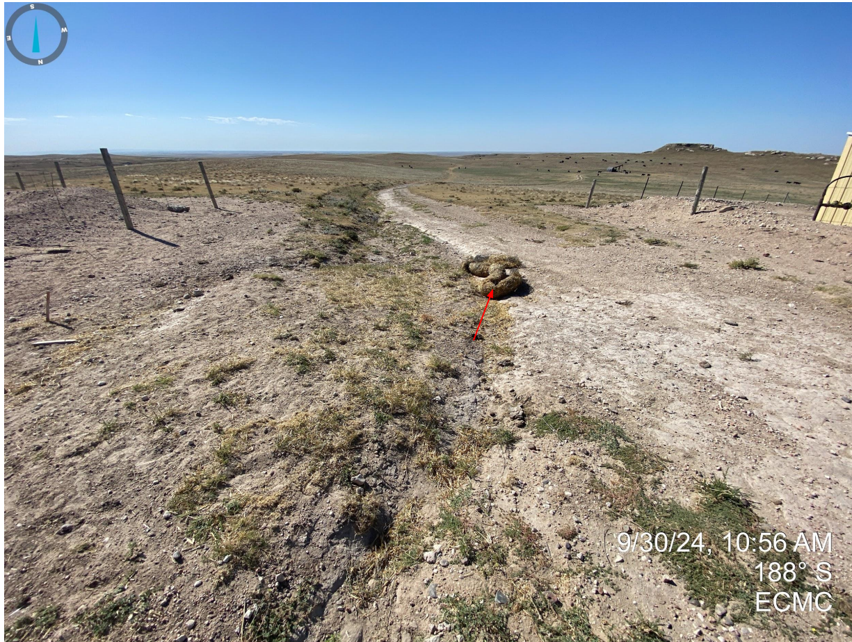
Photo 3. Erosion degradation along the access near production facilities. Straw wattles is now considered debris and needs to be removed.
