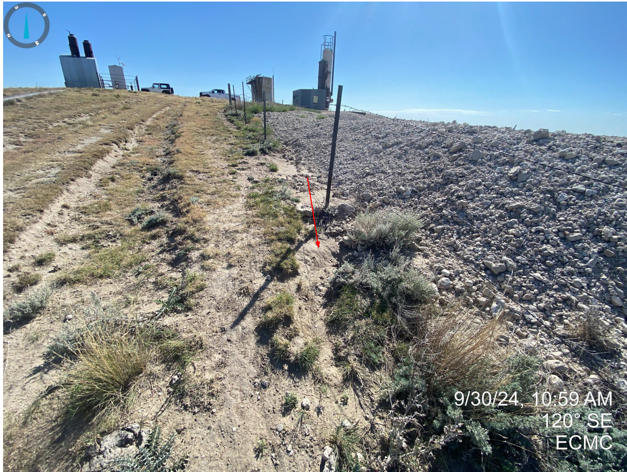
Photo 9. Erosion degradation on north side of pit.
