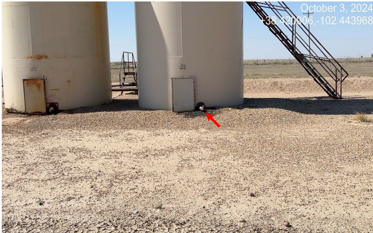
Photo 2. Facing west at the backside of the tank battery. The tank on the left appears to be rusted out on the bottom and the outlet at red arrow has oil stained soils.
