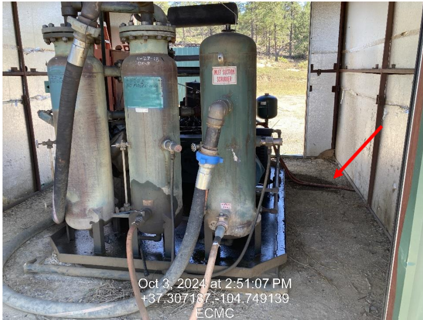
Photo 5 – Stained soils near day tank
