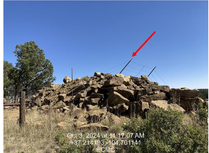
Photo 8 – Pit Fencing Inadequate
