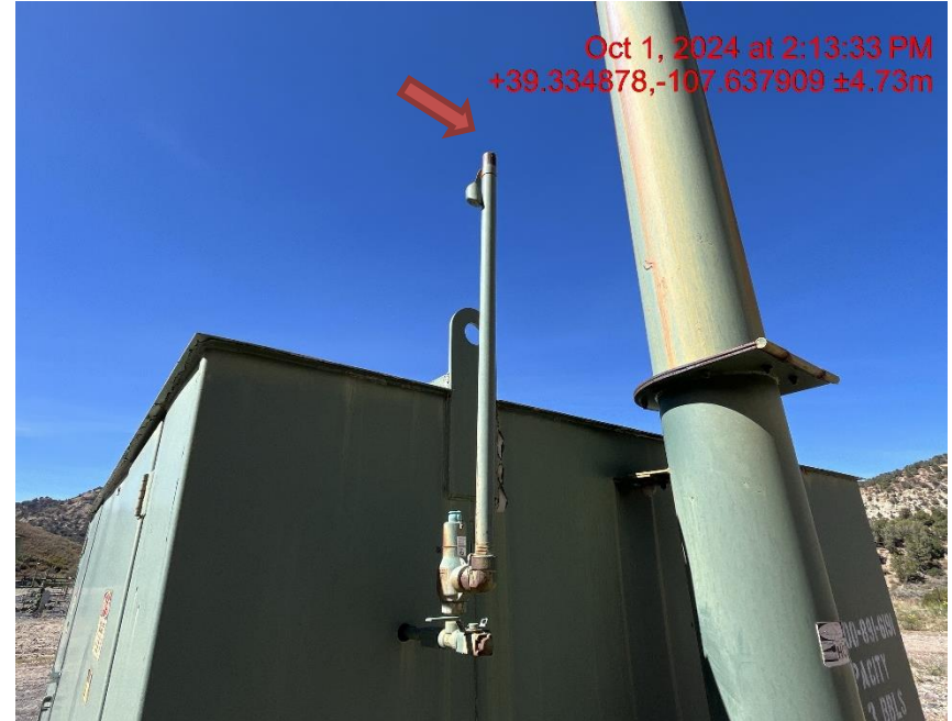
Photo # 6828 PRV vent line does not comply with CECMC pressure safety rules
