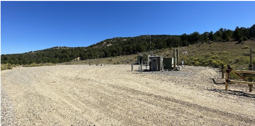
South West corner of location.
