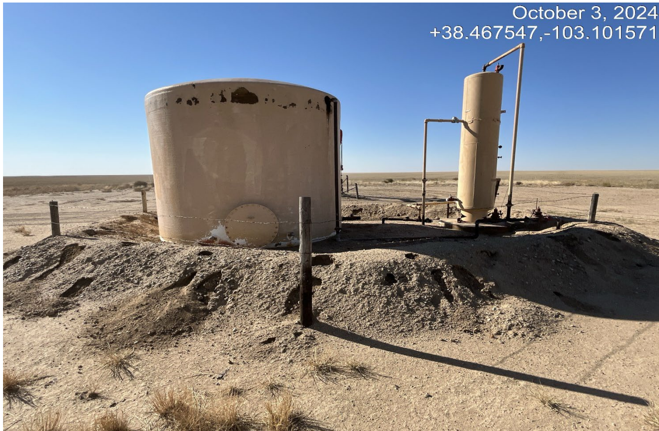
Photo 3. Facing toward the tank. The berm around the tank has been rebuilt. The sides of the berm are not compacted.
