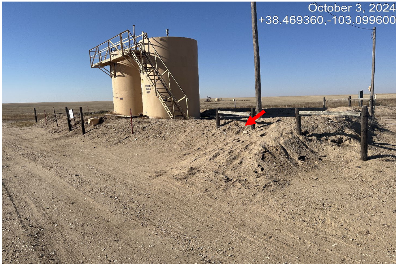
Photo 1. Facing toward the offsite tank battery location. The fence is not adequate to prevent livestock entry and there is no gate at the red arrow.
