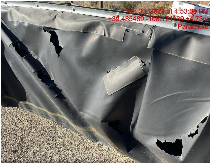
Holes in secondary containment liner - Photo #06641
