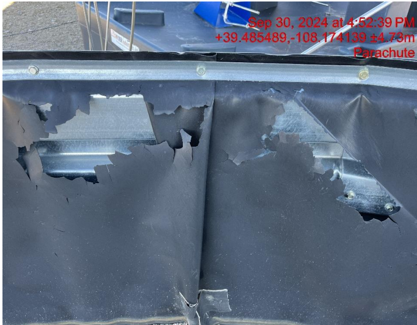
Holes in secondary containment liner - Photo #06639
