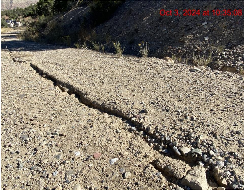
Rill Erosion on Access Road into Location – Photo #03865
