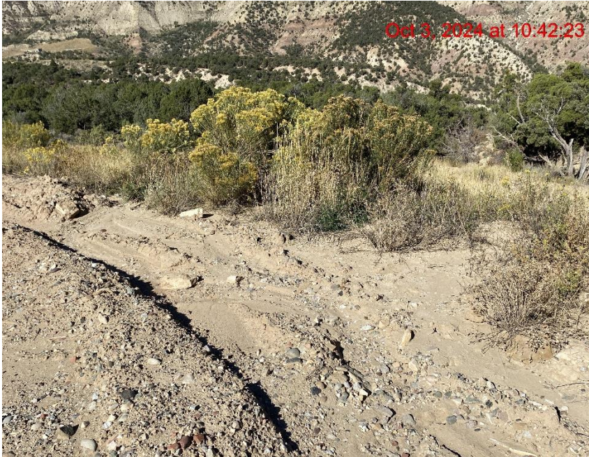
Rill Erosion from Access Road Transporting Sediment Offsite – Photo #03879
