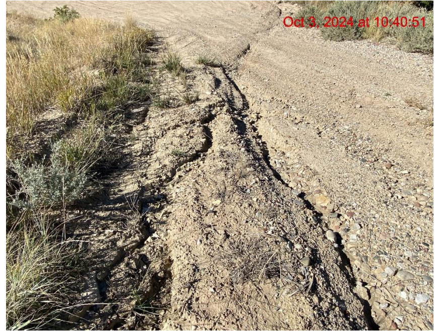
Rill Erosion on Access Road to Wellheads – Photo #03878
