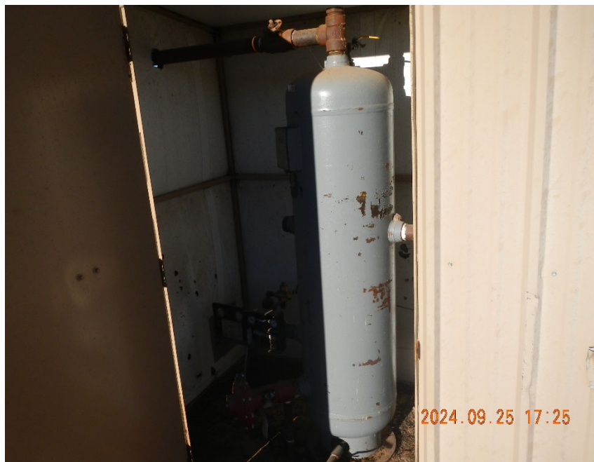
3. Vertical separator inside separator shed.
