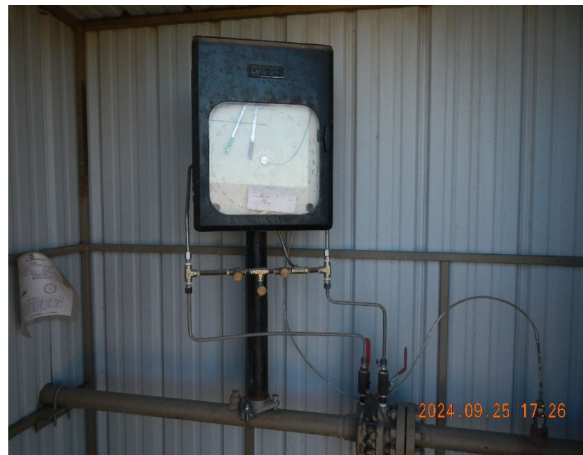
4. Gas meter inside meter shed.
