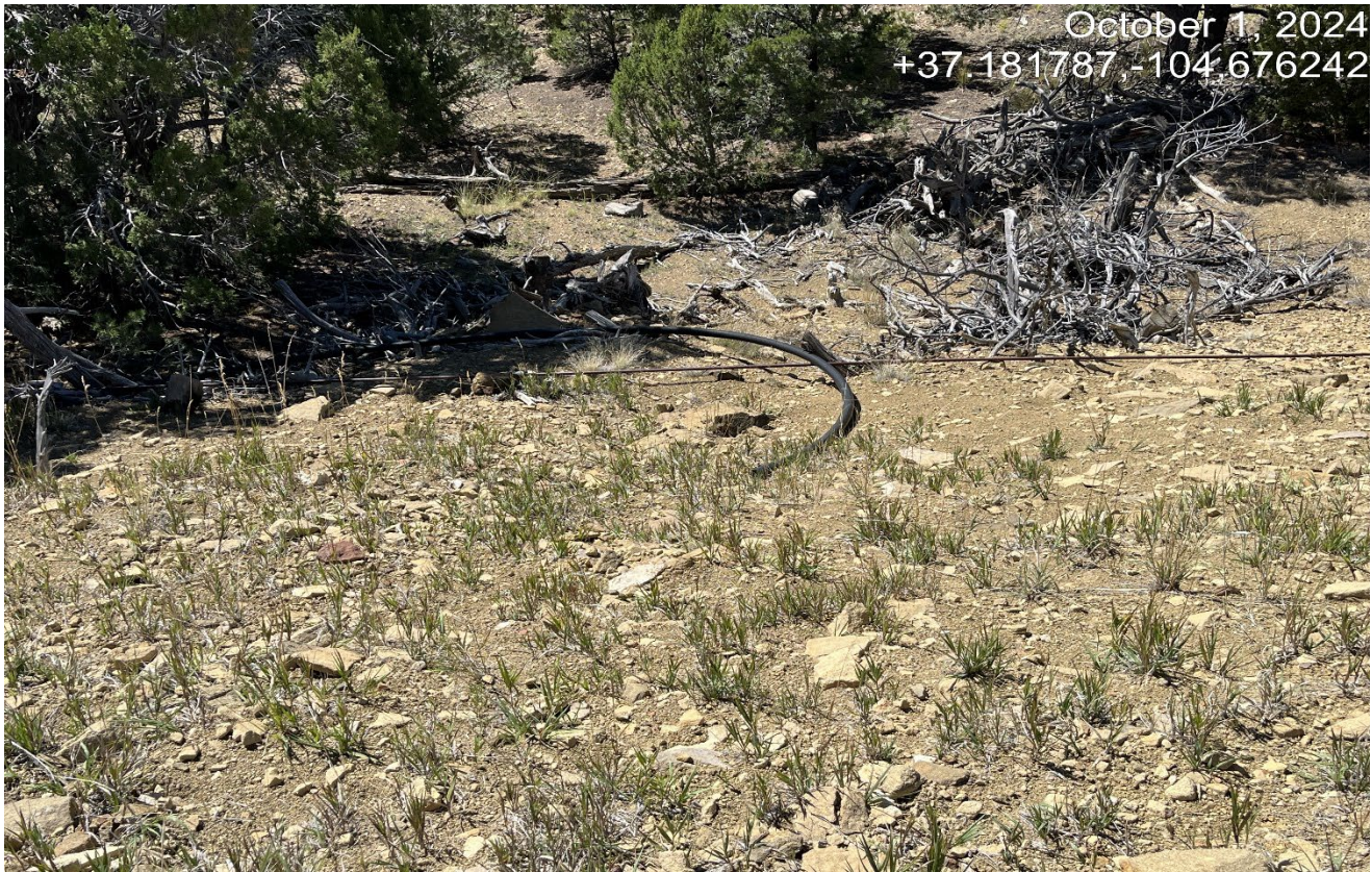
Photo 4. There is a plastic pipe and a steel rode at the bottom of the fill slope that needs to be removed.
