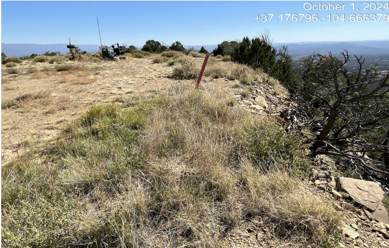
Photo 3. Facing southeast along the fill slope which appears to be stabilized.
