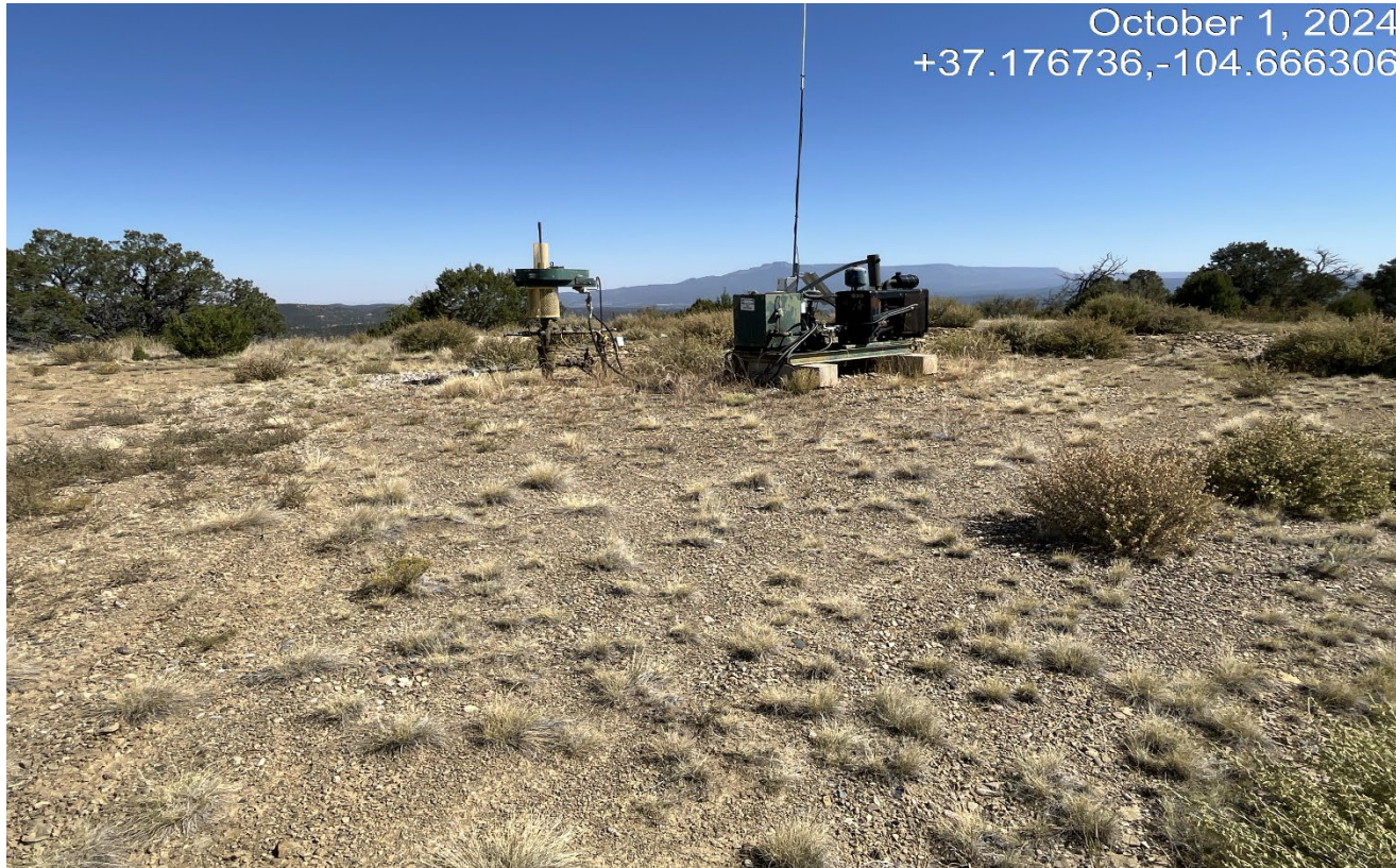
Photo 1. Facing east toward the wellsite.
