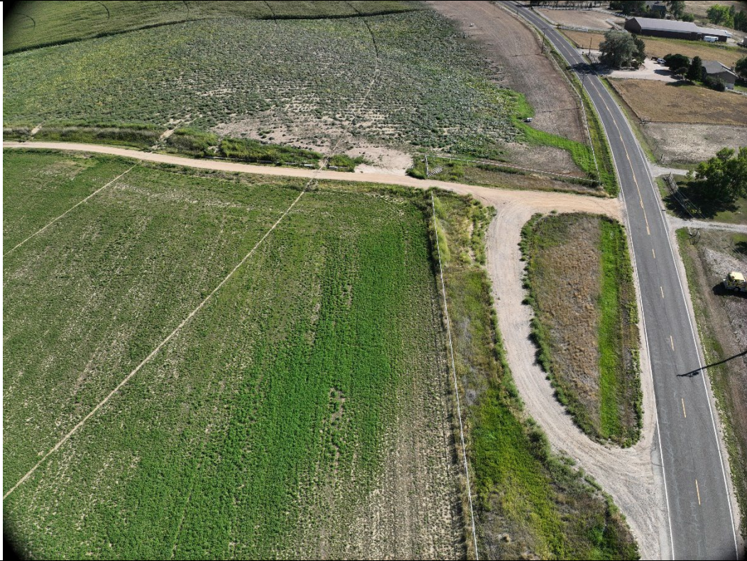
In View – Tank Battery, Flowline
