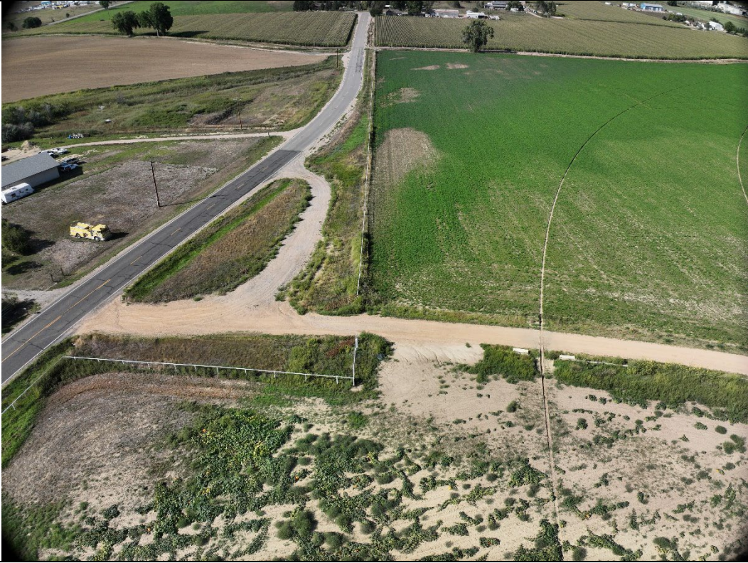
In View – Tank Battery, Flowline
