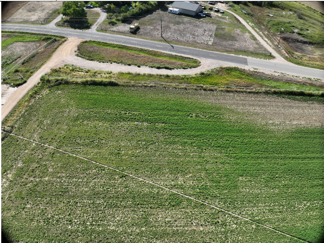
In View – Tank Battery, Flowline
