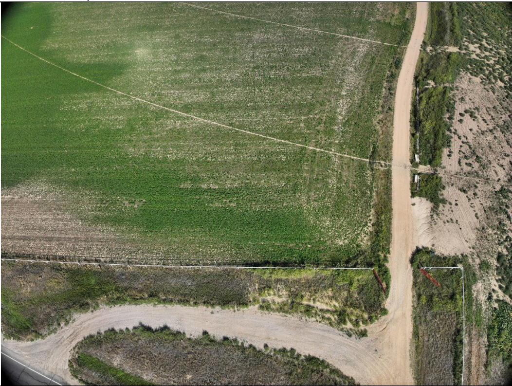
In View – Tank Battery, Flowline
