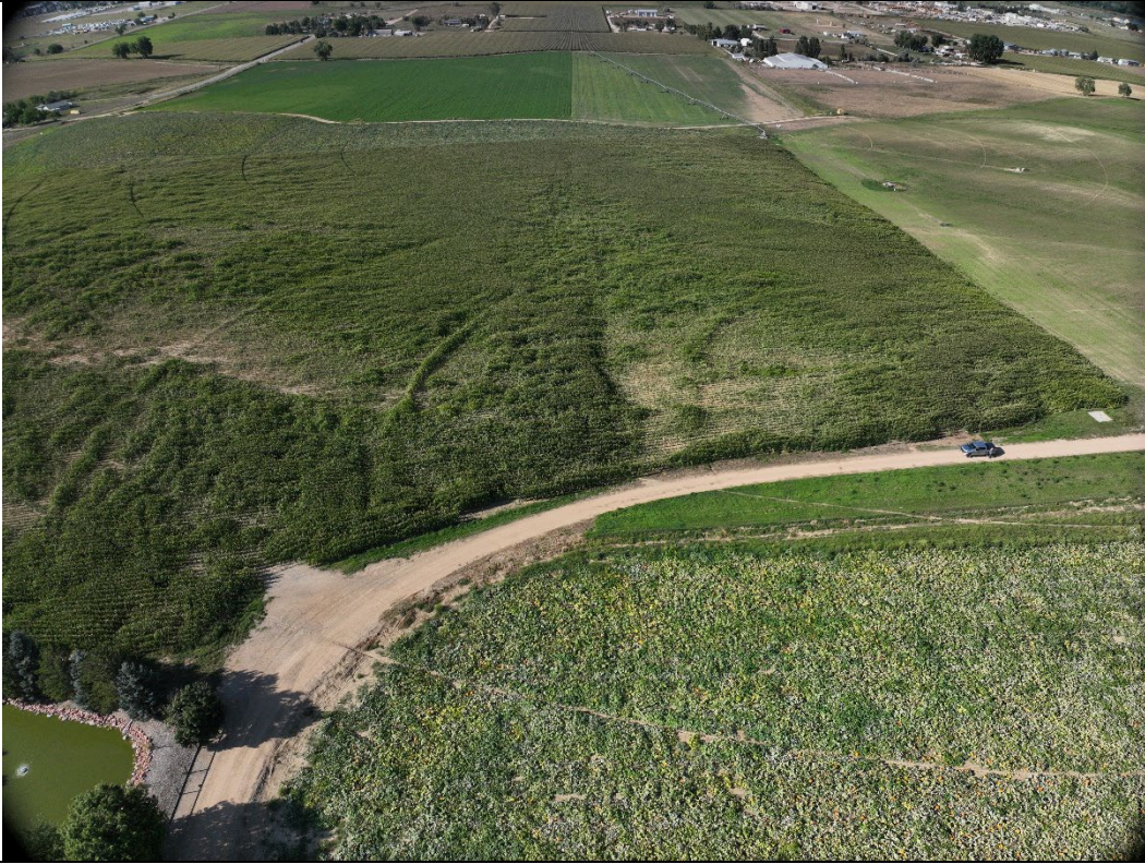
In View – Well, Tank Battery, Access Road, Flowline
