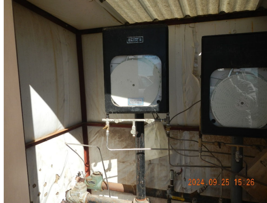
4. Gas meter inside remote meter shed.
