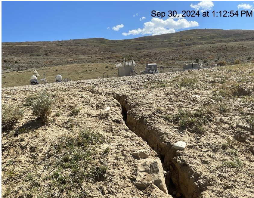
Photo # 2887 Erosion & transport of sediment off location
