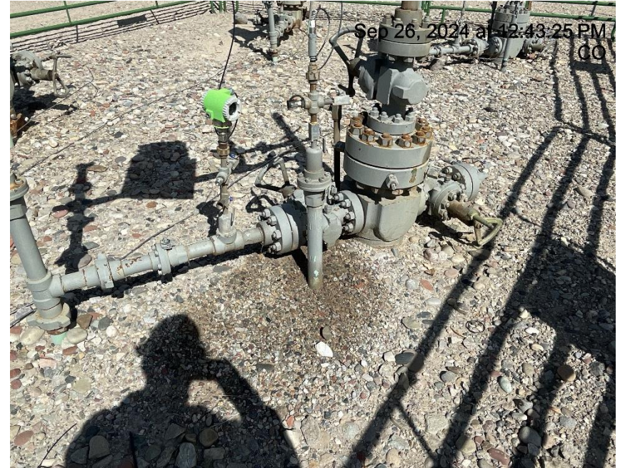
Photo # 2129 Staining near wellhead
