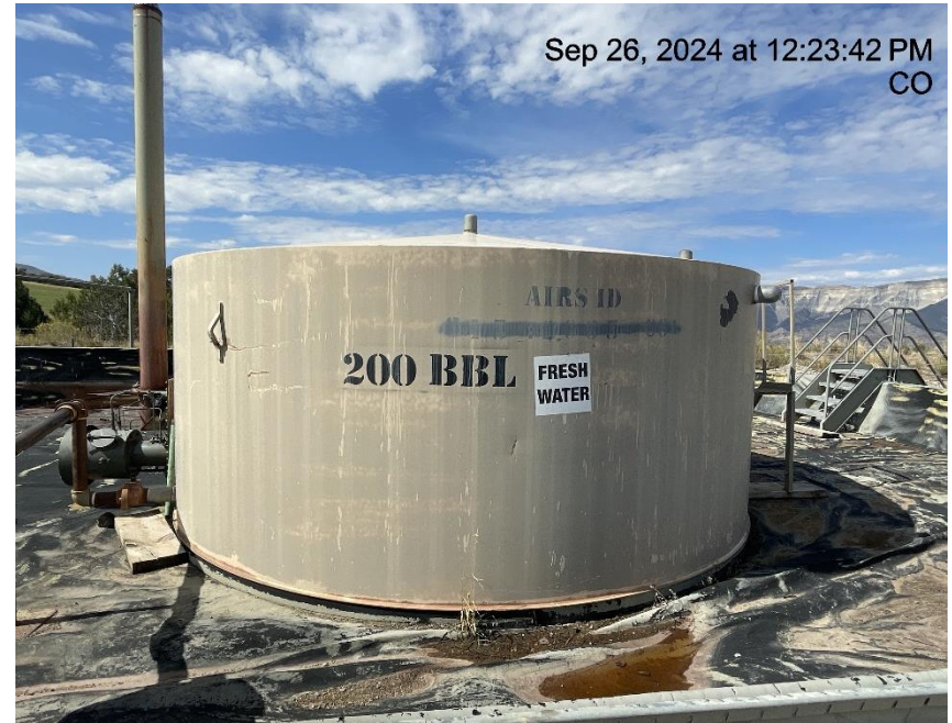
Photo # 2127 Tank lacks required labeling
