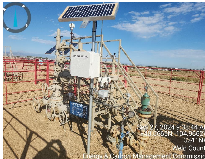
Photo 2 well head and equipment
