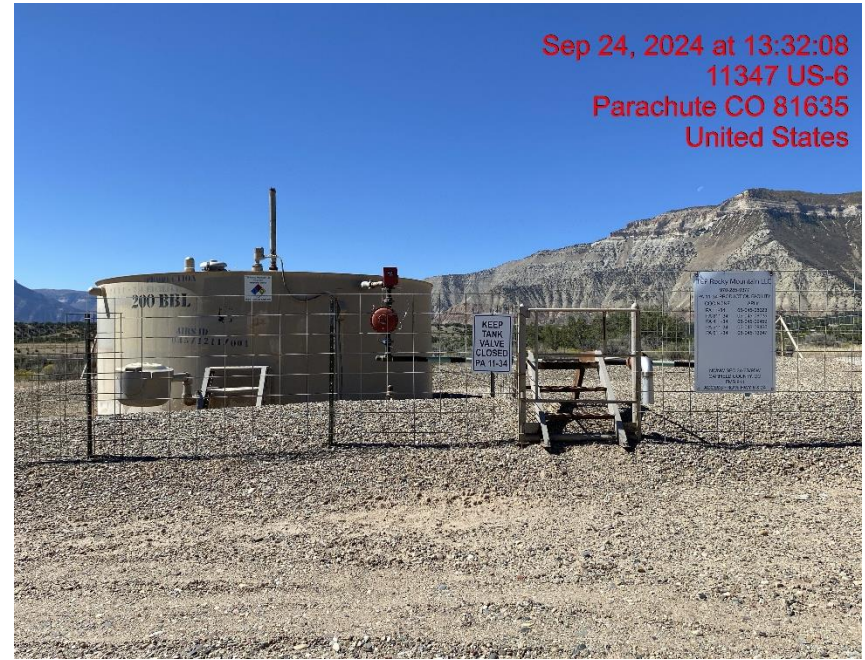
Tank Battery – Photo #03669
