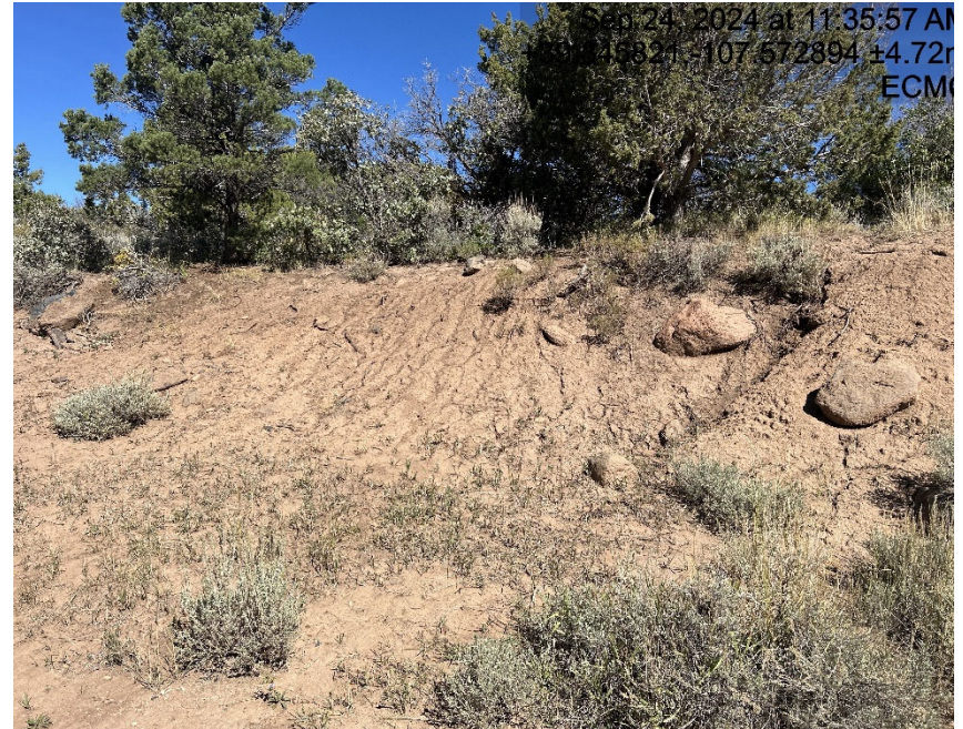
Erosion on cut slope
