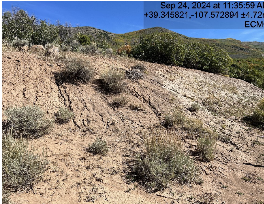
Erosion on cut slope
