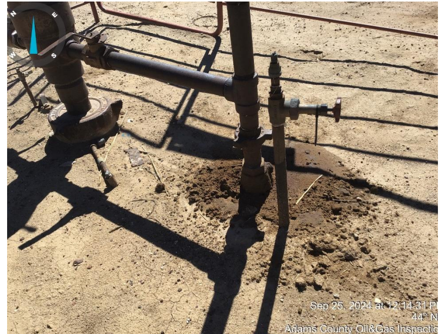
Photo#2 Stained soil around ground valve at wellhead
