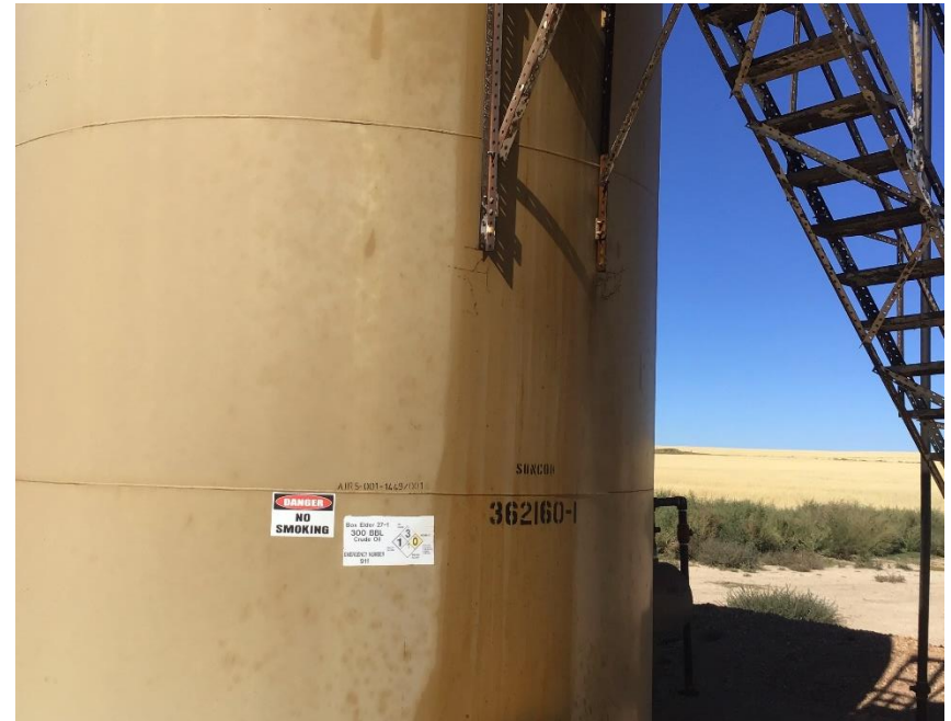
Photo#6 Oil appears to be leaking from thief hatch going down the side of the production tank
