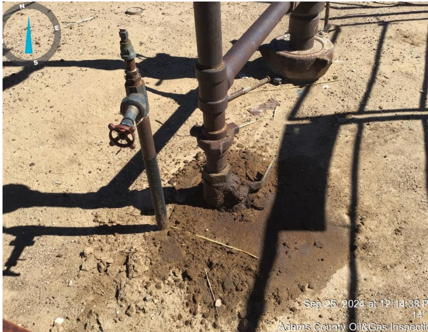
Photo#3 Stained soil around ground valve at wellhead
