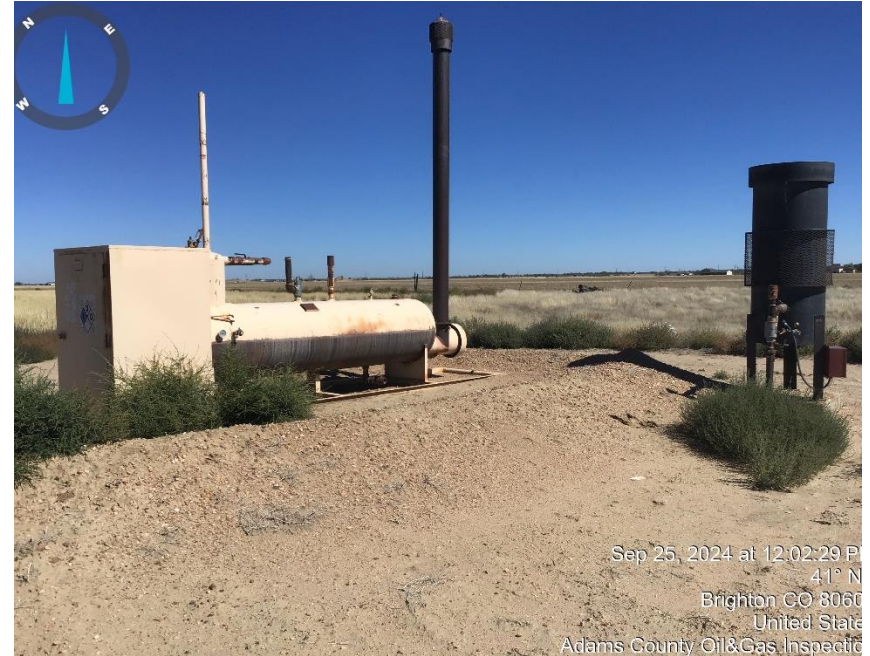
Photo#2 Separator/ECD
