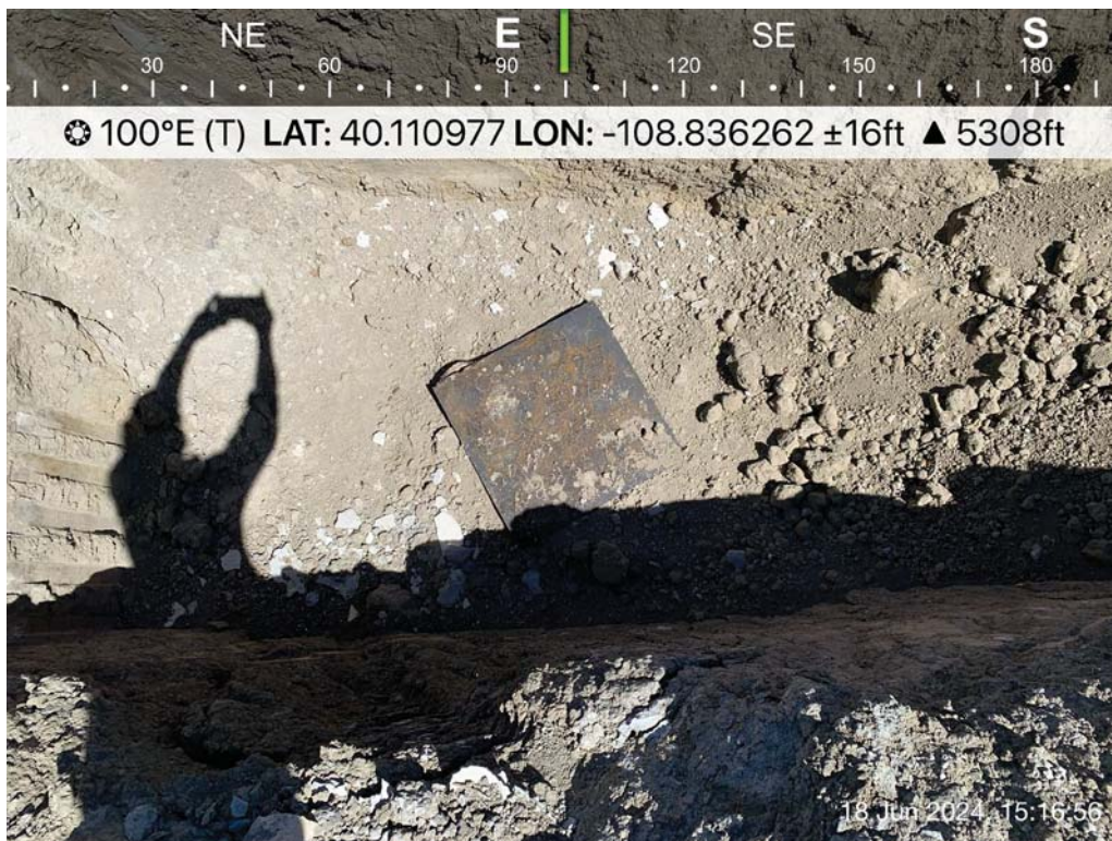
Photo 1: Calup #14 (OWP) P&A wellhead, no methane detected, view from above.
