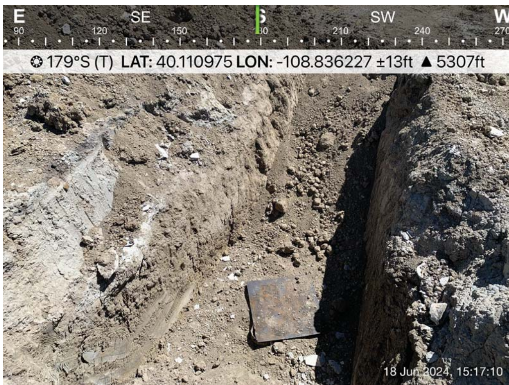
Photo 4: Calup #14 (OWP) P&A wellhead, no methane detected, view south.
