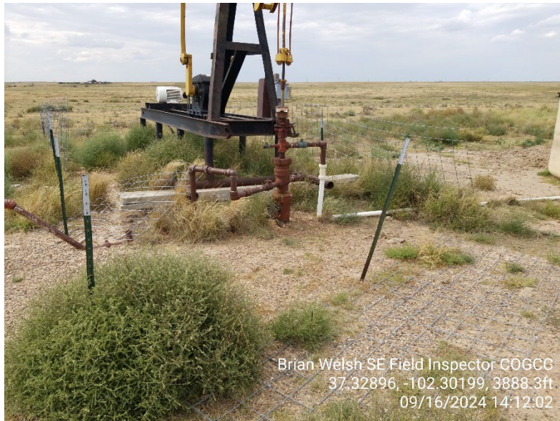
3. Wellhead and water leg. Fencing laying on the ground
