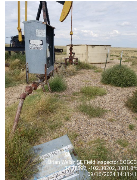
4. Meter run door laying on the ground. Lease sign isn't legible
